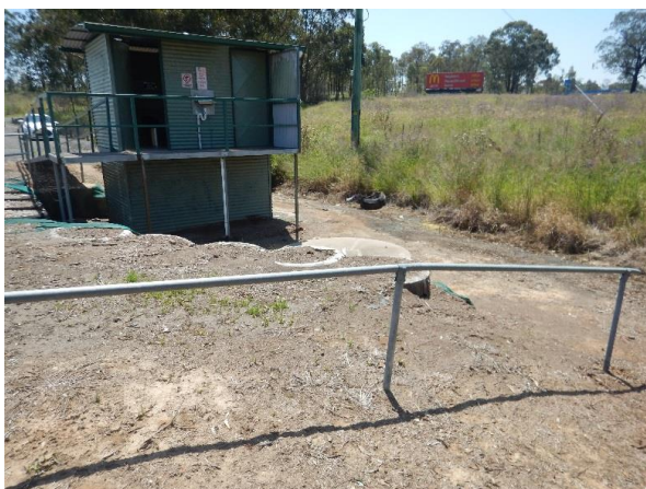
Figure 28: Toilet block in the rest area.
