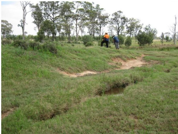
Figure 48: Dam on the main watercourse.
