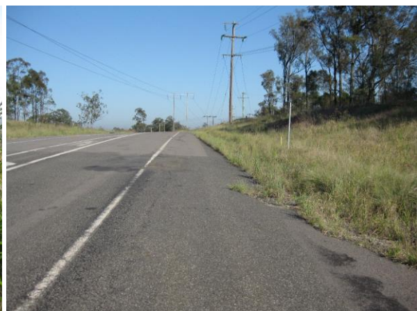
Figure 23: Former Golden Highway alignment.
