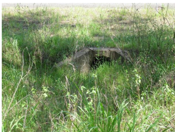
Figure 43: Culvert under the eastern section of former alignment.
