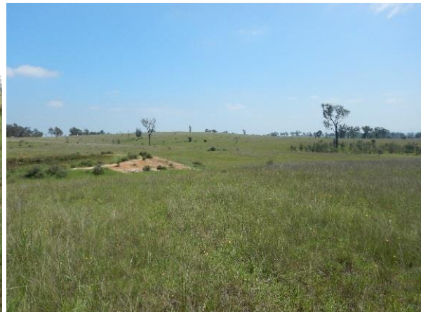
Figure 49: Dam on the minor watercourse.
