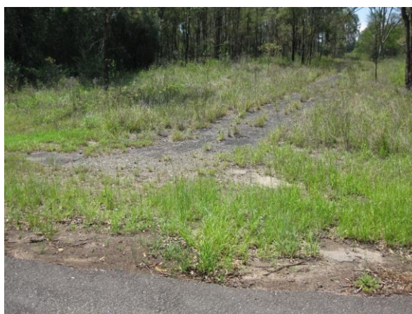
Figure 44: Road between the eastern section of former alignment and the highway.
