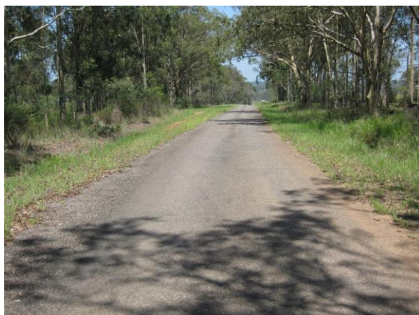
Figure 41: Eastern section of former alignment.
