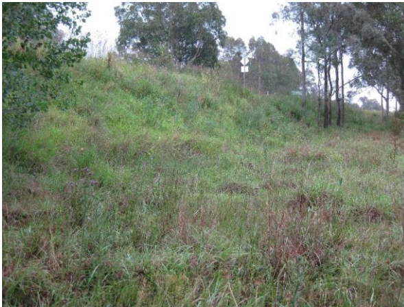
Figure 31: Embankment for the New England Highway.
