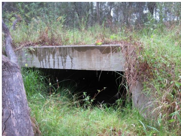
Figure 39: Culvert on the western section of former alignment.
