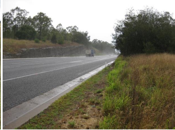
Figure 30: Cutting on the New England Highway.
