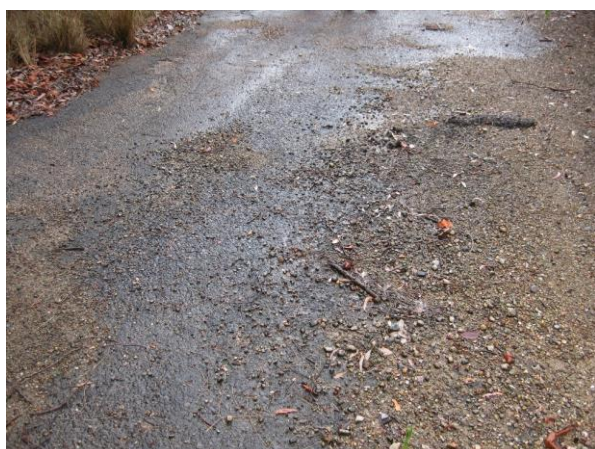
Figure 37: Road pavement on the western section of former alignment.
