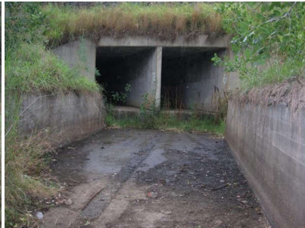
Figure 32: Culvert under the New England Highway.
