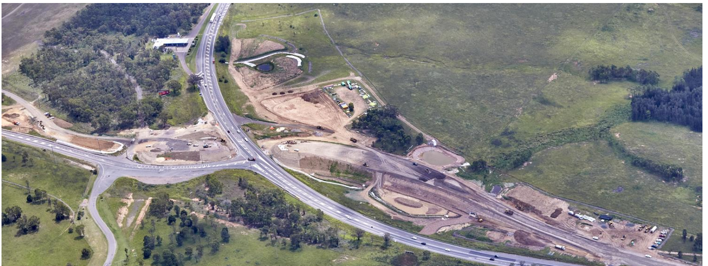
Aerial image of work progress
