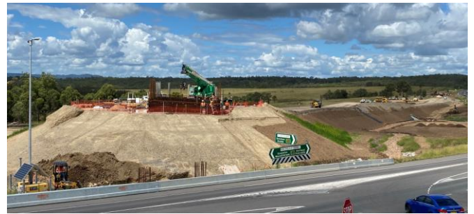
Construction at Golden Highway intersection
