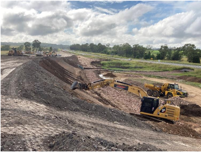
Fill placement and topsoiling
