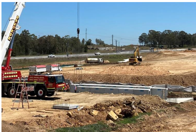
New culvert being built near the Golden Highway intersection
