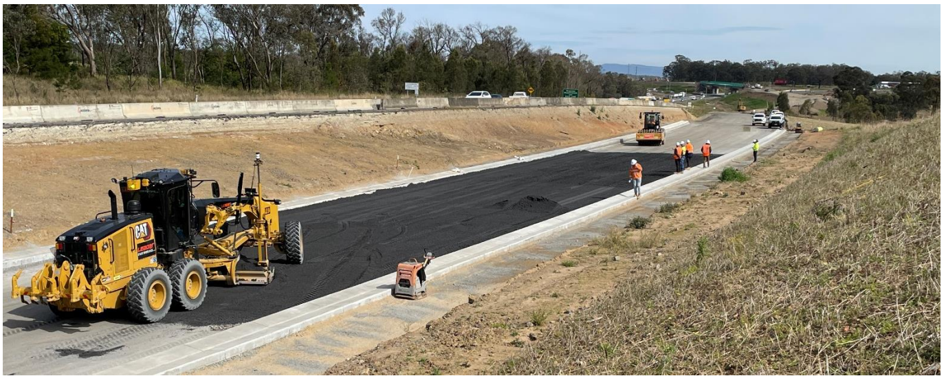
New eastbound lanes on the New England Highway under construction
