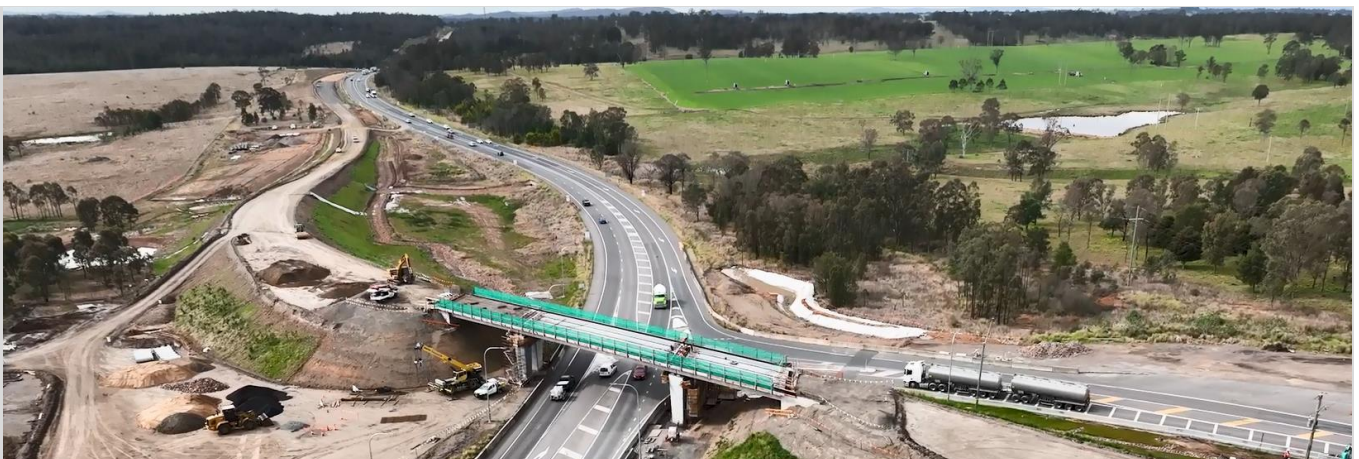
Aerial shot of the flyover bridge under construction
