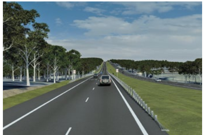
Artist impression: New England Highway, new divided road heading east towards Maitland
