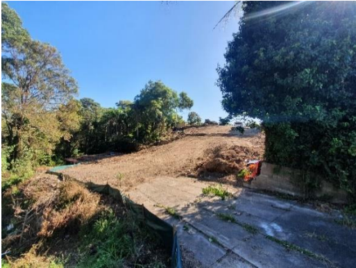
Image 1: Lookout Road house demolition
