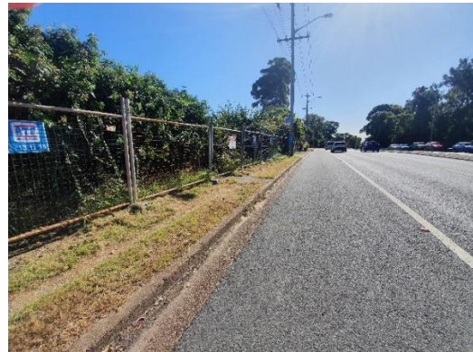
Image 2: Lookout Road house demolition
