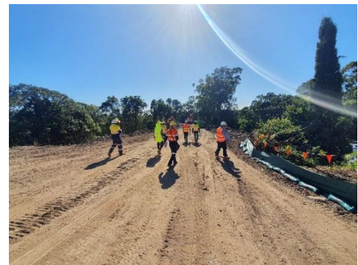
Image 4: Lookout Road house demolition
