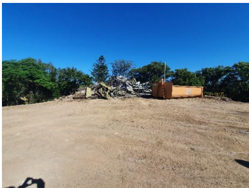
Image 3: Lookout Road house demolition
