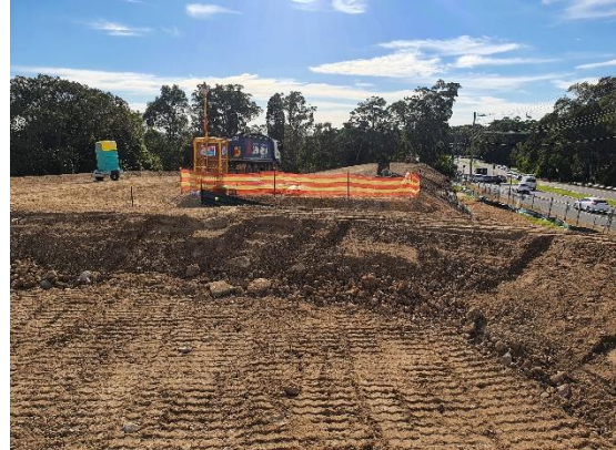
Image 4: Lookout Road house demolition
