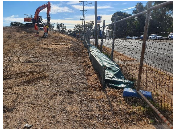
Image 2: Lookout Road house demolition
