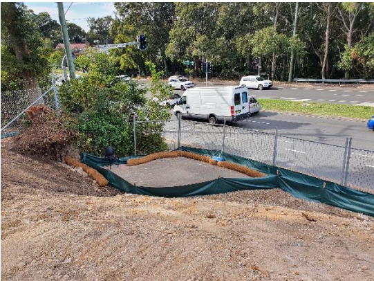
Image 5: Lookout Road house demolition
