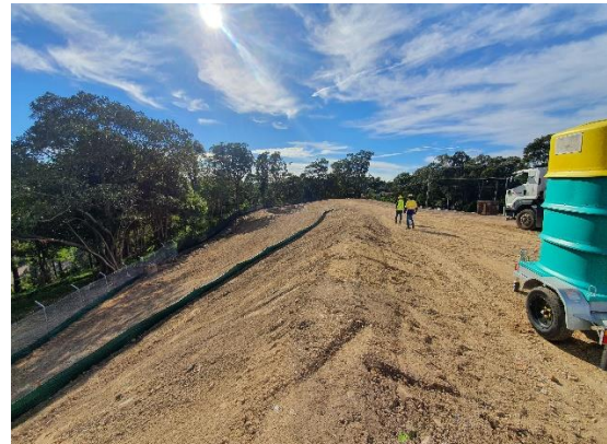
Image 6: Lookout Road house demolition
