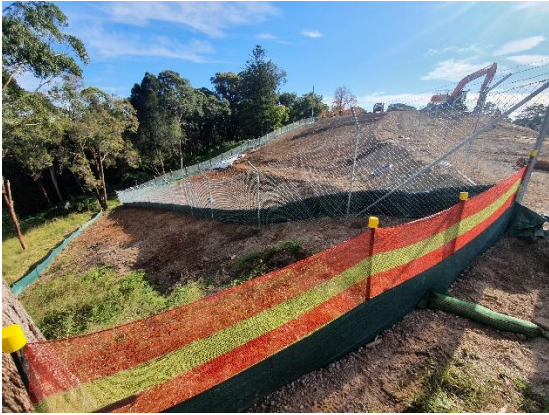
Image 1: Lookout Road house demolition
