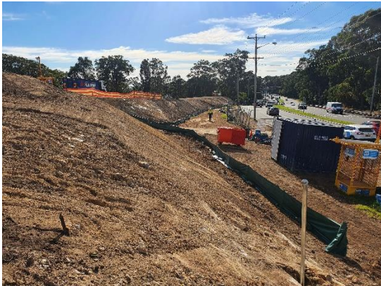
Image 3: Lookout Road house demolition
