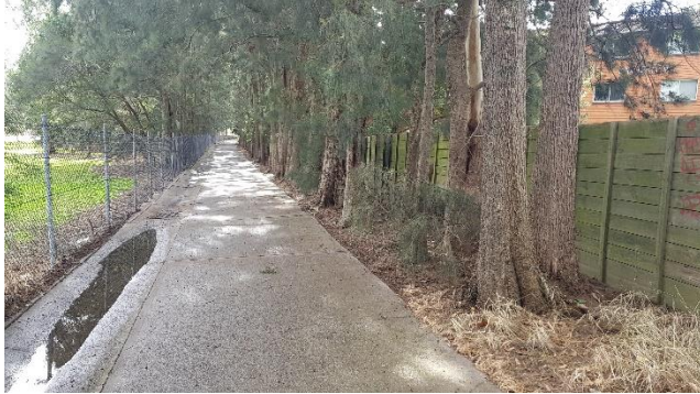
Photo 1: Pedestrian and bike path adjacent to Main Road, Jesmond
