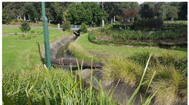
Photo 6: Jesmond Park, left of drain is location of Ancillary Facility D
