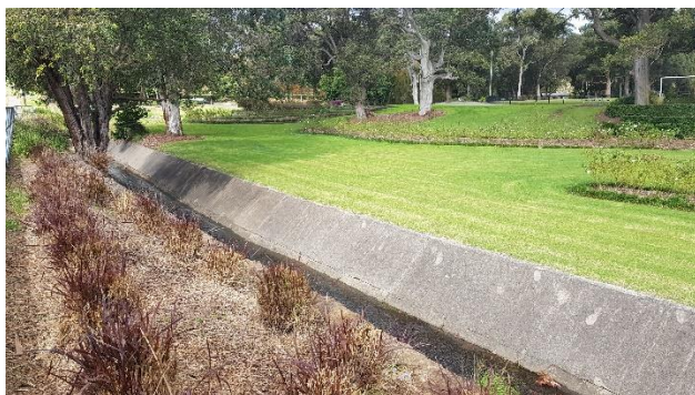
Photo 5: Jesmond Park, Looking towards Ancillary Facility D
