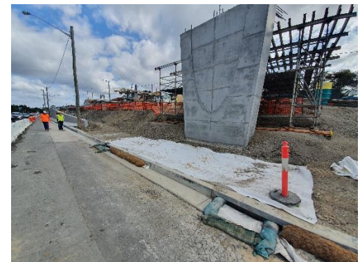
Image 6: Northern Bridge Pier, Newcastle Road
