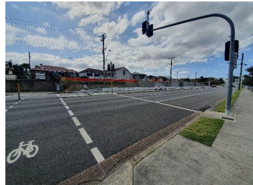
Image 4: Retaining Wall, Newcastle Road (1)
