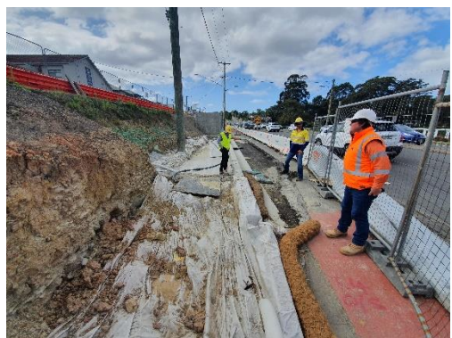
Image 5: Retaining Wall, Newcastle Road (2)
