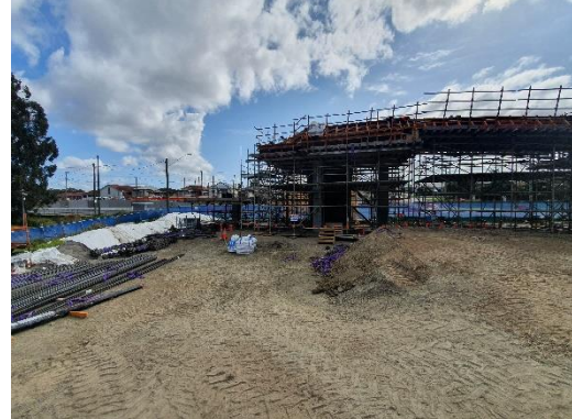
Image 2: Southern Bridge Pier, Newcastle Road
