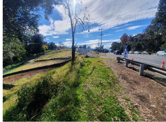
Image 2: Utility Relocation Works
