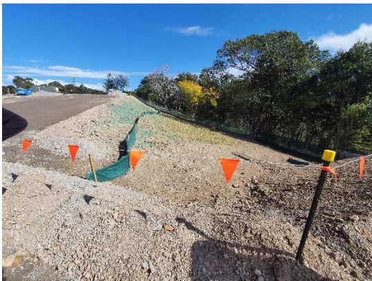
Image 5: Utility Relocation Works
