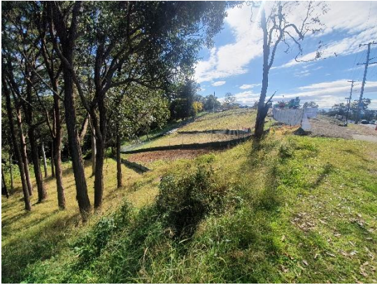
Image 1: Utility Relocation Works
