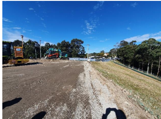
Image 6: Utility Relocation Works
