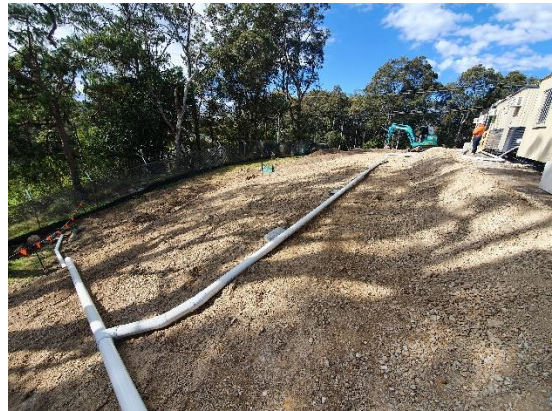
Image 4: Utility Relocation Works
