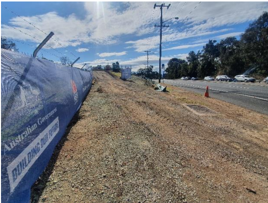
Image 3: Utility Relocation Works
