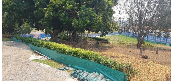
Photo 2: ERSED controls, tree removal and barrier fencing
