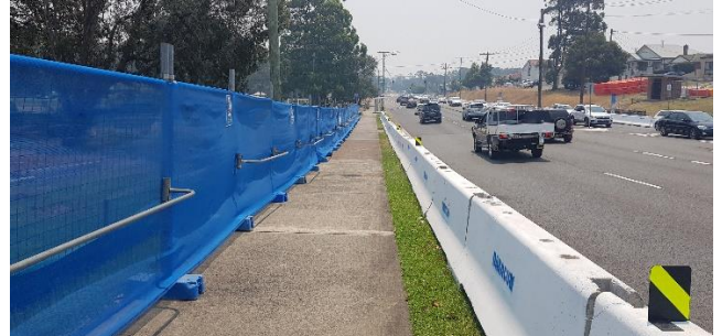
Photo 4: Barrier fencing and pedestrian barrier on Newcastle Road
