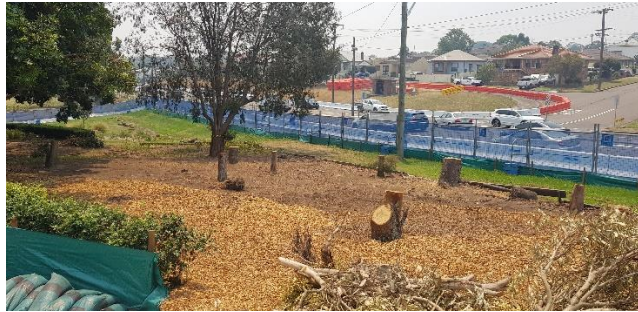
Photo 1: tree removal and barrier fencing
