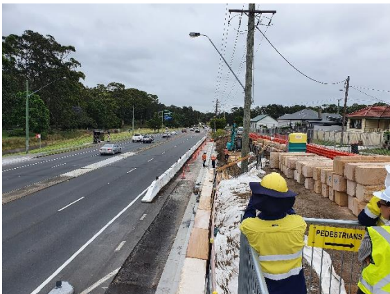
Image 5: Northside of SPB (looking West)
