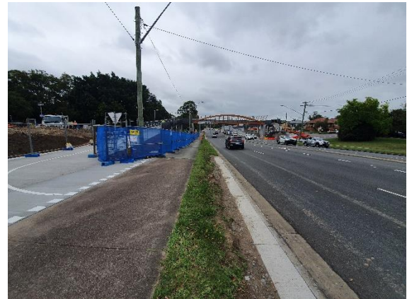
Image 4: Newcastle Road (looking West)
