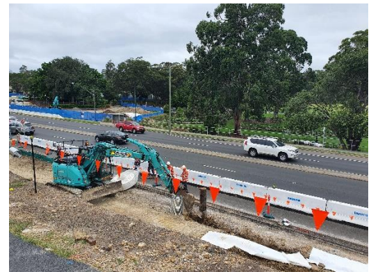
Photo 4: Newcastle Road works (1)
