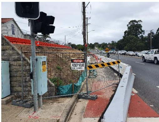
Photo 3: View looking east along Newcastle Road
