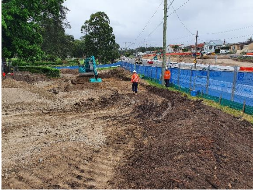
Photo 1: Piling pad construction
