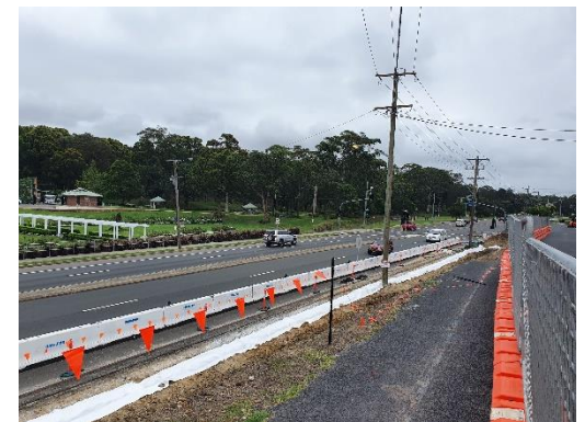
Photo 6: Newcastle Road works (3)
