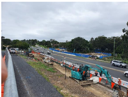
Photo 5: Newcastle Road works (2)
