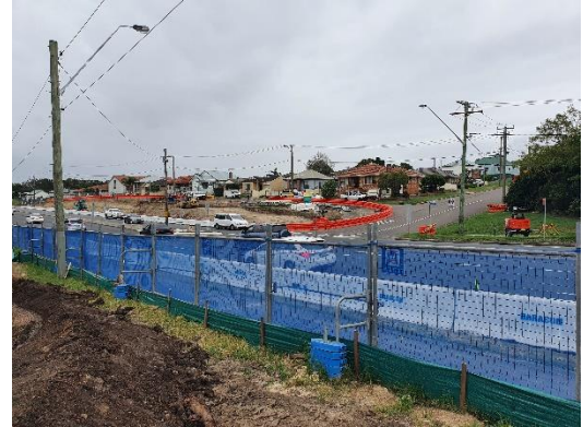
Photo 2: View across Newcastle Road towards Coles Street
