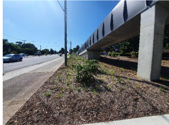
Image 2: Southside SPB entry and landscaping
