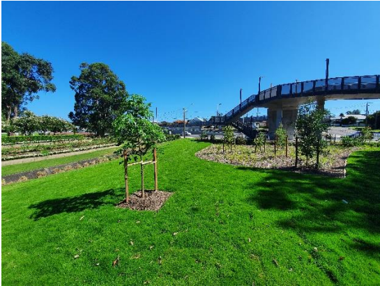
Image 1: SPB, Jesmond Park looking west
