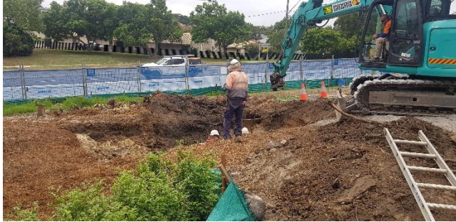
Photo 1: tree removal and utilities work
