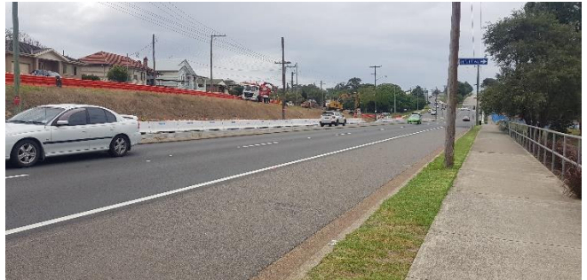
Photo 4: Newcastle Road site works
