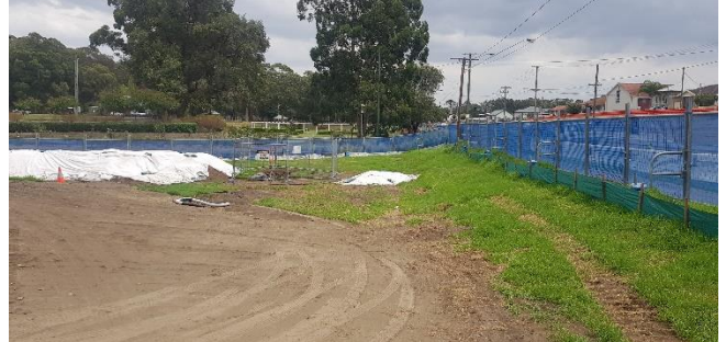
Photo 2: utilities works – water main.
