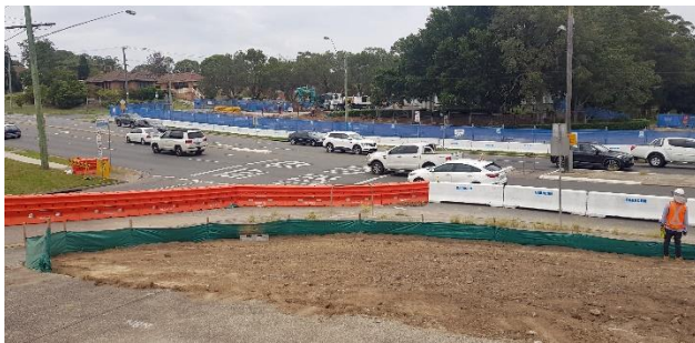
Photo 5: Steel Street / Newcastle Road intersection
