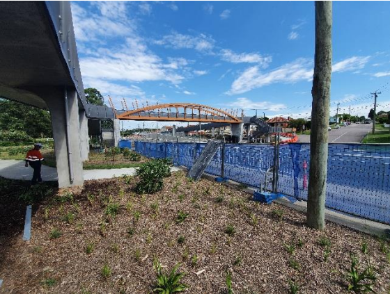
Image 3: SPB and access ramp (southside)
