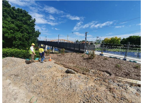
Image 2: Southside SPB entry and landscaping
