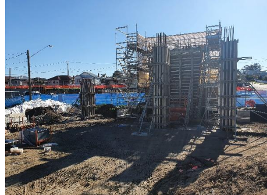
Image 2: Southern Bridge Pier
