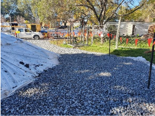
Image 1: Project Site, Cnr of Newcastle Road and Robinson Avenue
