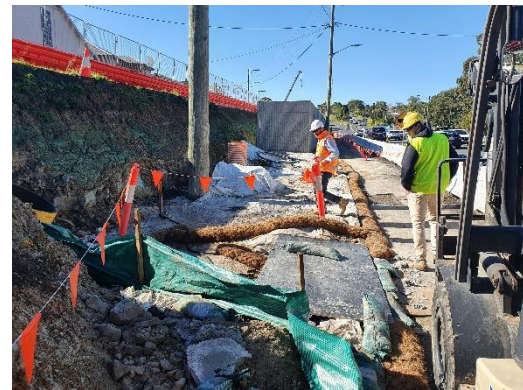
Image 4: Retaining Wall, Newcastle Road (2)
