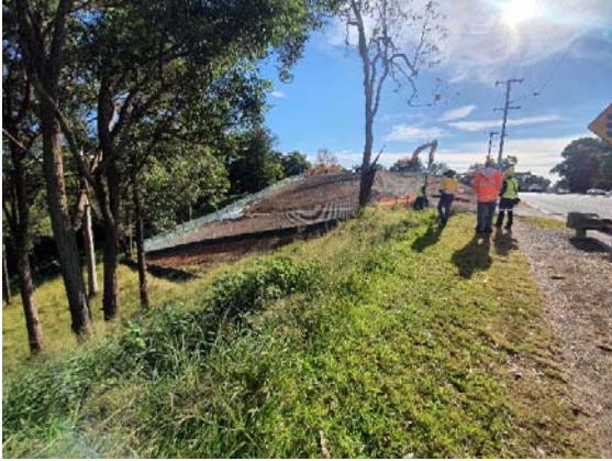
Image 1: Lookout Road house demolition
