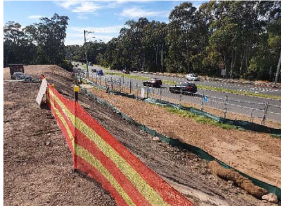
Image 6: Lookout Road house demolition
