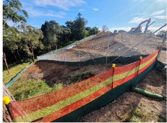
Image 2: Lookout Road house demolition
