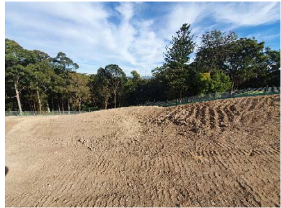
Image 4: Lookout Road house demolition
