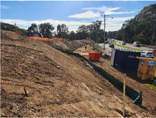
Image 3: Lookout Road house demolition
