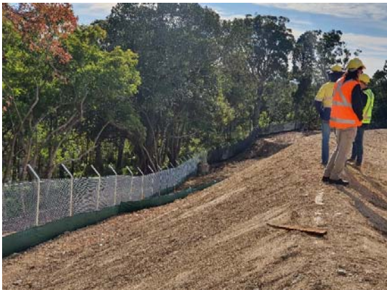
Image 5: Lookout Road house demolition
