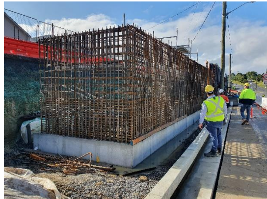
Image 4: Retaining Wall, Newcastle Road (2)
