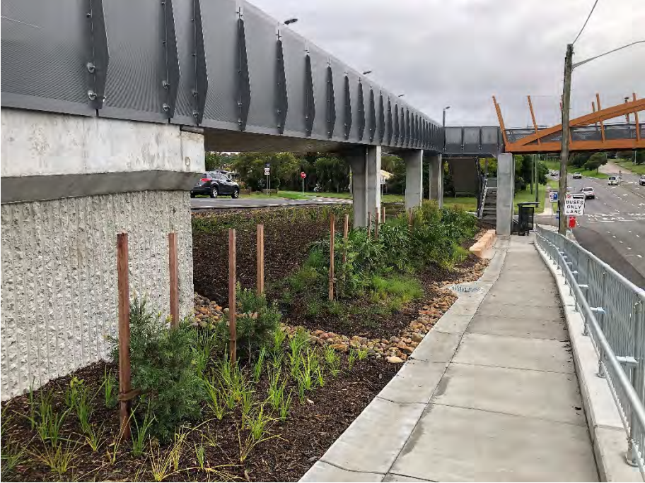
Photograph D.6 View of completed bridge along Newcastle Road (east)
