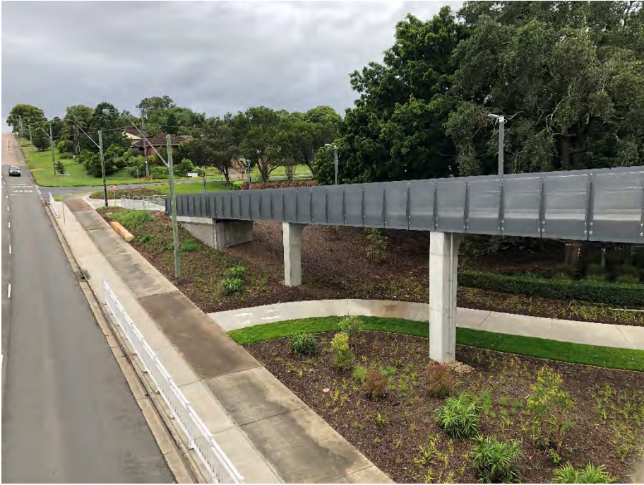
Photograph D.3 Completed revegetation around pedestrian footbridge
