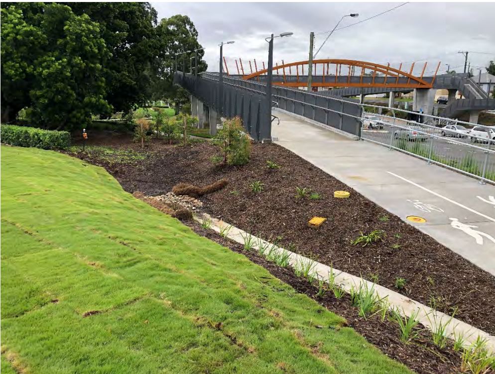
Photograph D.2 Completed revegetation around pedestrian Footbridge
