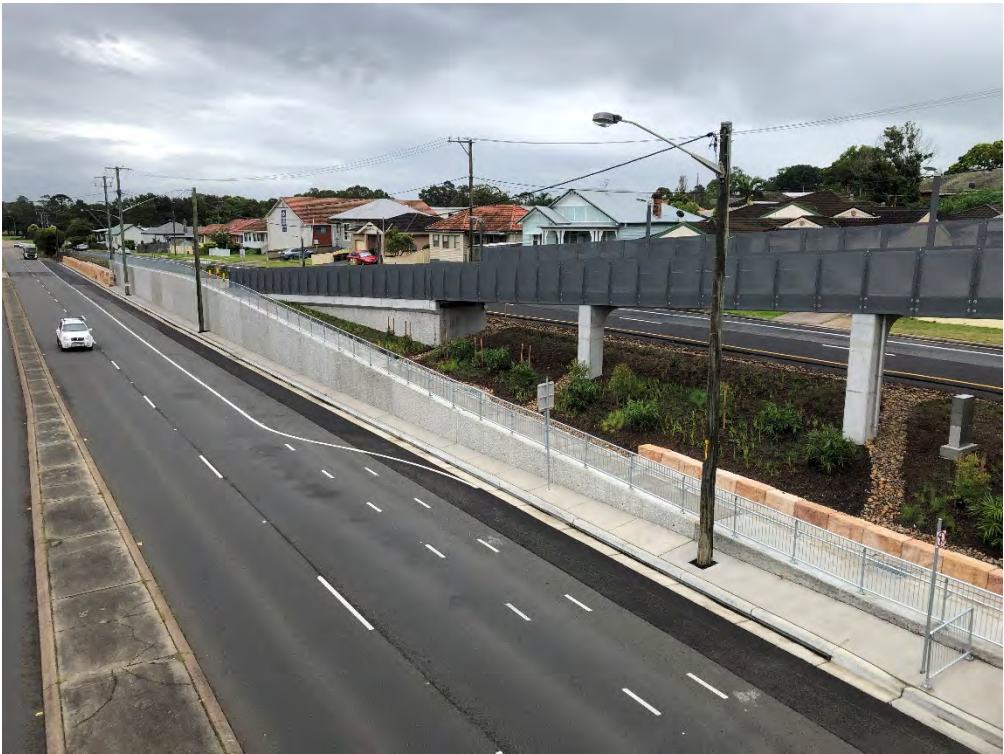
Photograph D.4 Completed footbridge (northern side)
