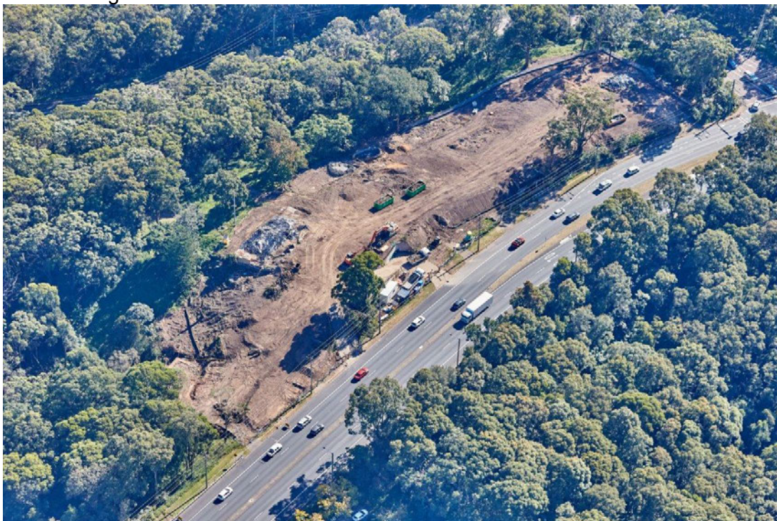
Figure 2 house demolition work
