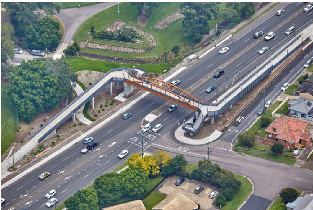
Figure 3: Stage 2 Shared Path Bridge
