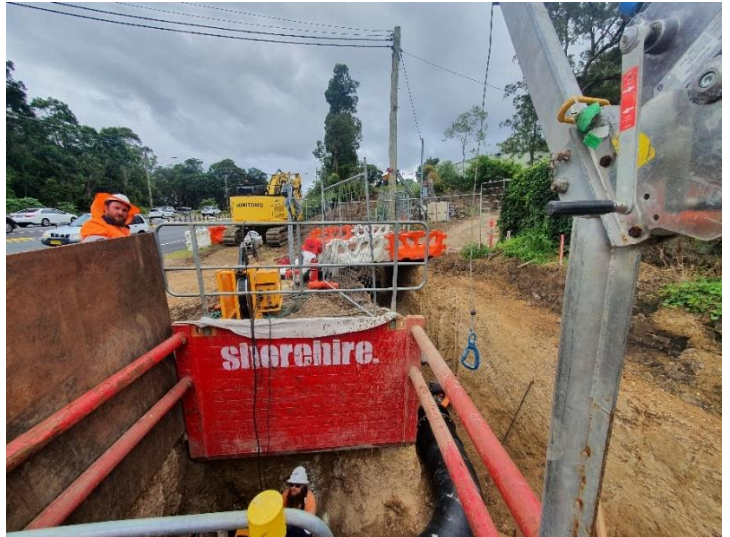
Image 4: Utility relocation works
