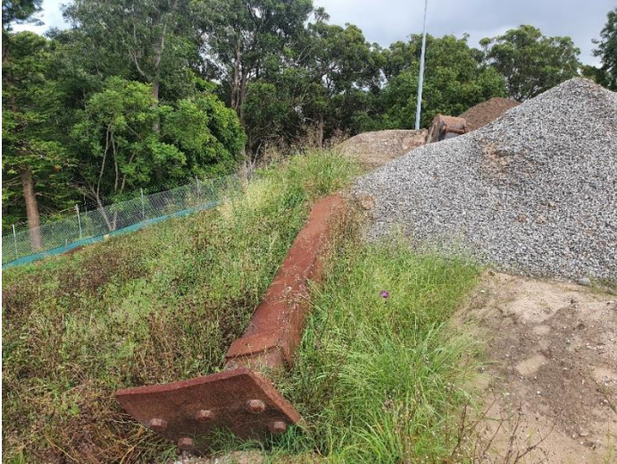
Image 1: Utilities relocation works
