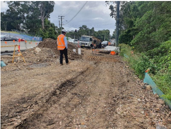
Image 7: Utility relocation works
