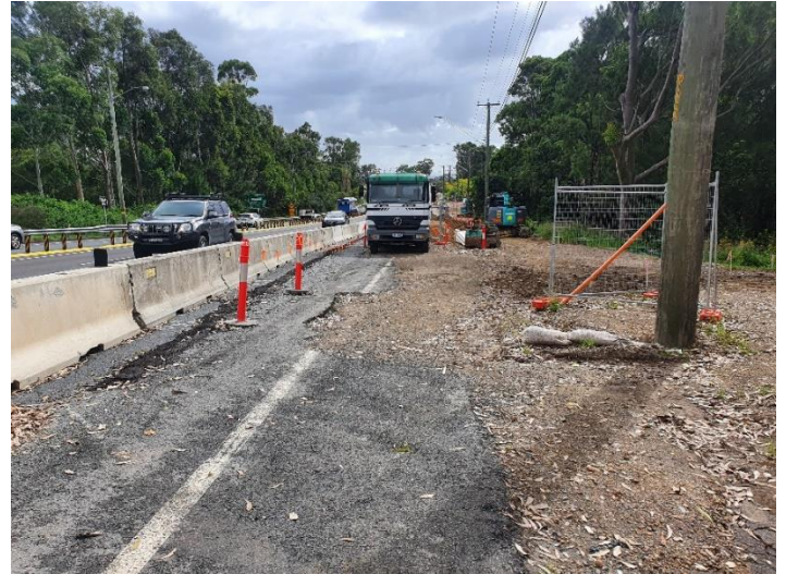
Image 6: Utility relocation works
