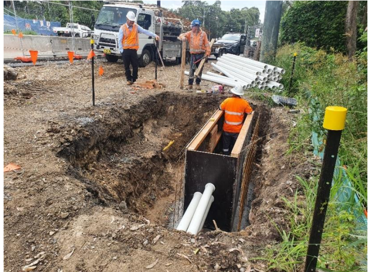
Image 8: Utility relocation works
