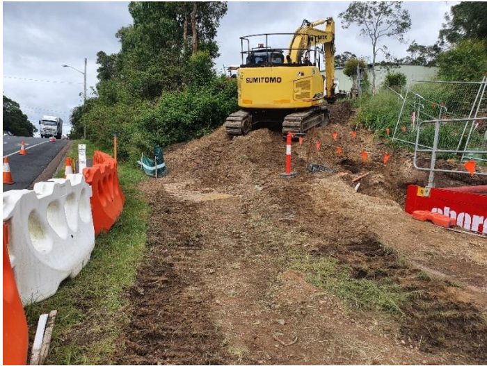
Image 5: Utility relocation works
