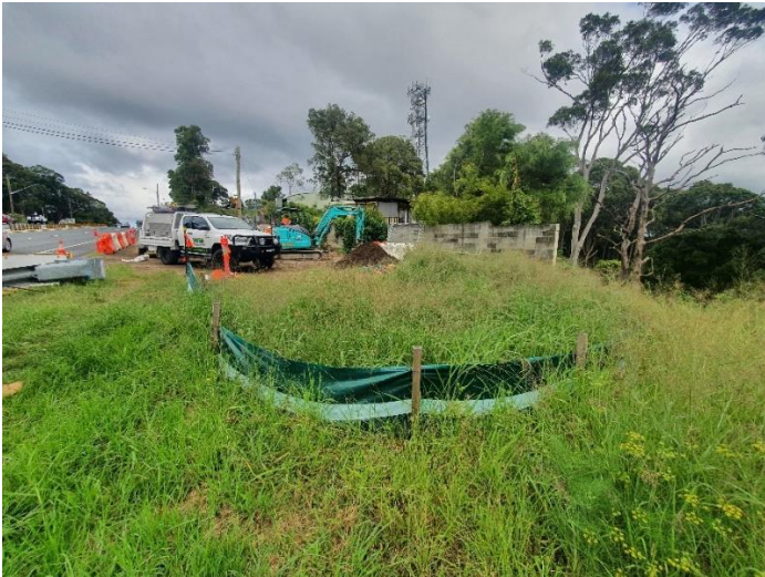
Image 3: Utility relocation works
