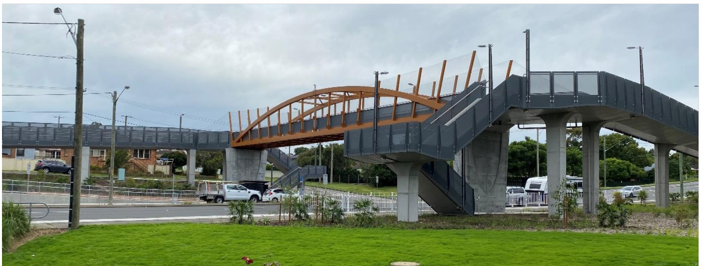
Completed shared path bridge over Newcastle Road.
