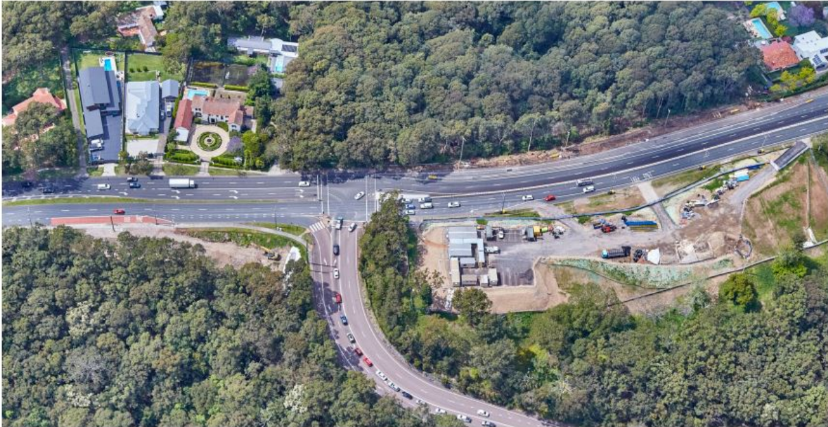
Figure 4.2: Southern Utilities - Lookout Road
