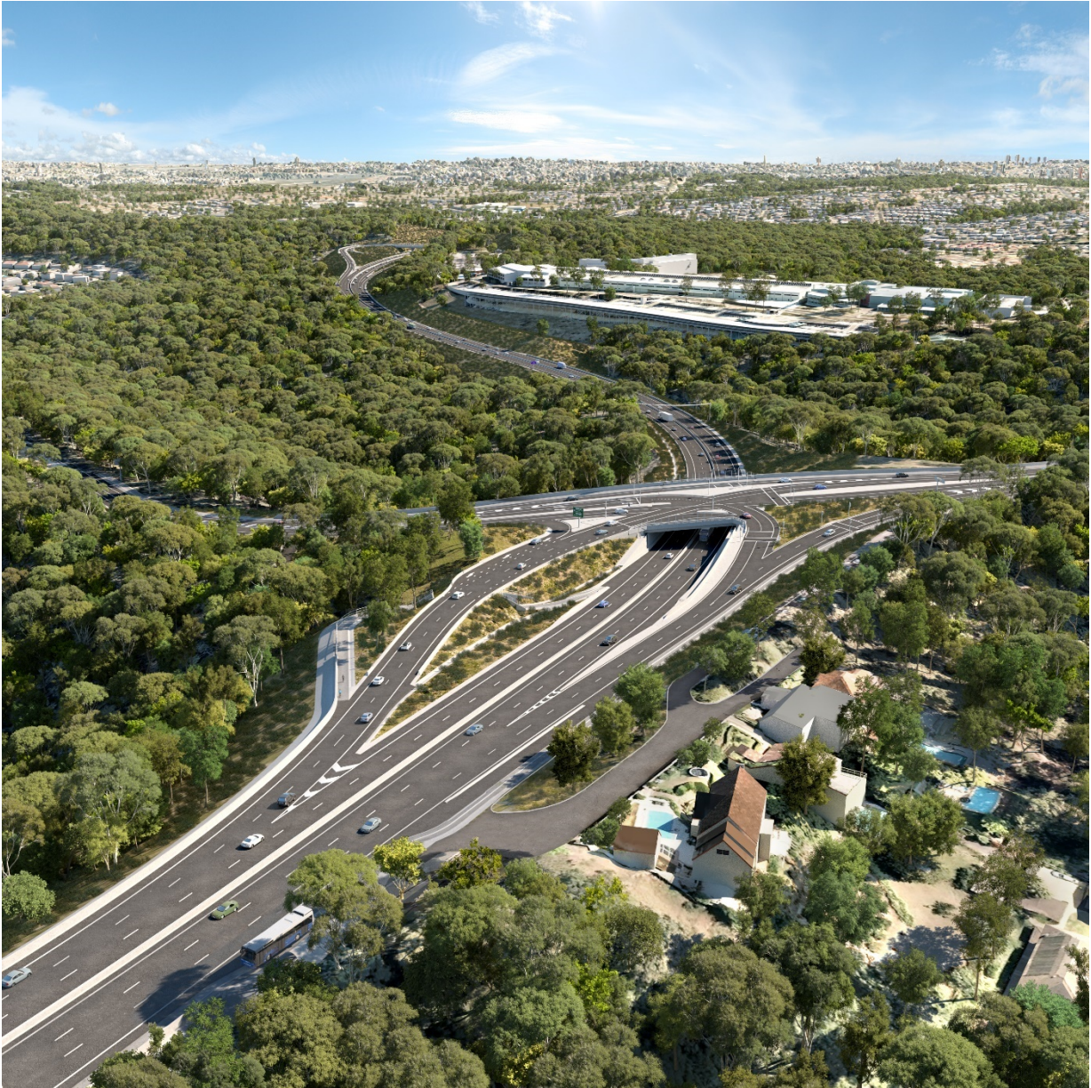
Figure 1.3: The Project – southern interchange
