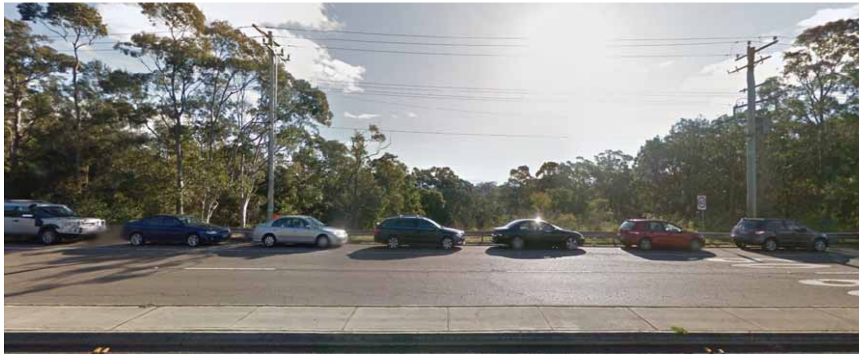
Figure 7.4 View from Lookout Road looking west towards the project. (Source: Google Street View)
