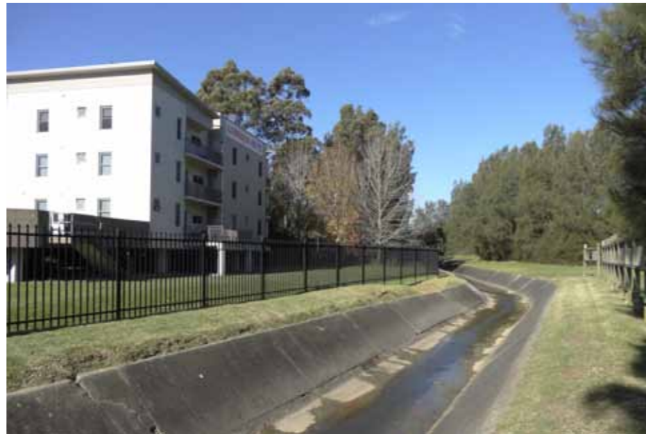
Figure 3.68 An apartment complex defines the southeast corner of this zone and interfaces with the existing Inner Newcastle Bypass and Jesmond Interchange. Note the Casuarinas to the right of the photograph providing effective screening to the interchange.
