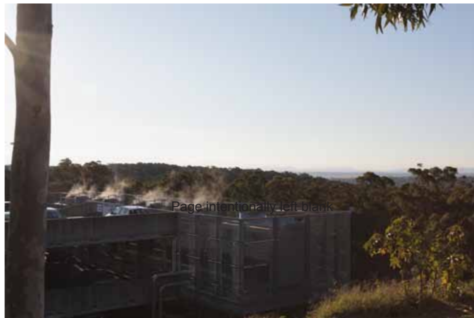
Figure 2.1 View looking west across the bushland setting from the Hospital Precinct carpark
