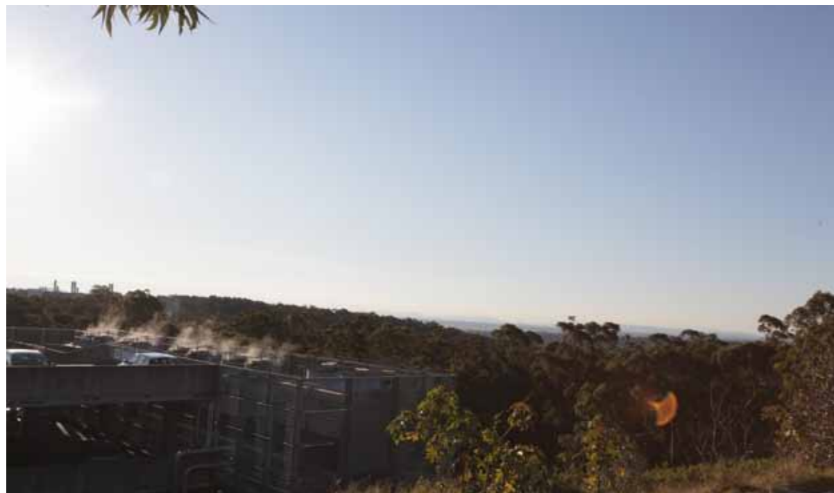
Figure 7.10 View from Jacaranda Drive within the Hospital Precinct looking west towards the project.
