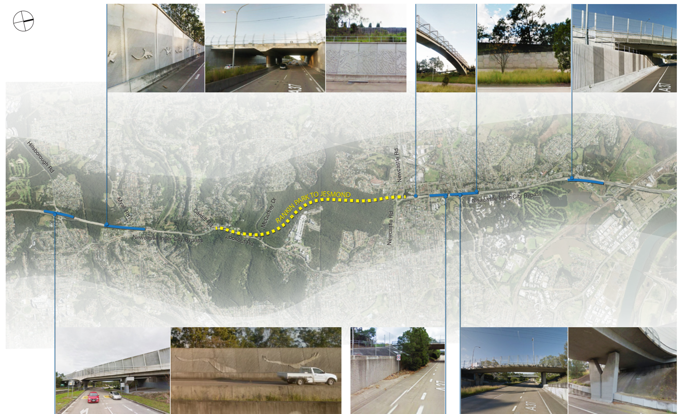
Figure 2.20 A number of distinctive treatments and themes have been applied to built form elements along the overall bypass, leading to some visual discontinuity between the various sections of the roadway.
