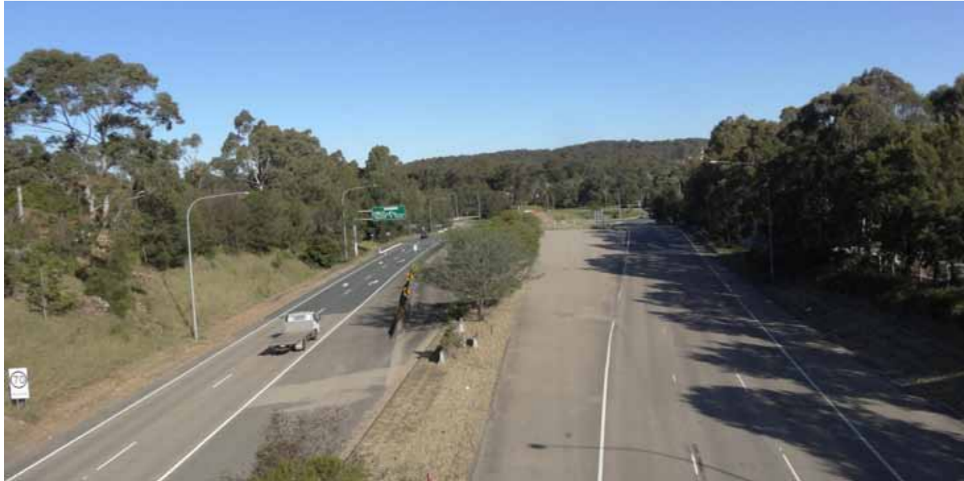
Figure 7.26 View from the pedestrian overpass across the bypass at Jesmond looking south, north of Newcastle Road.
