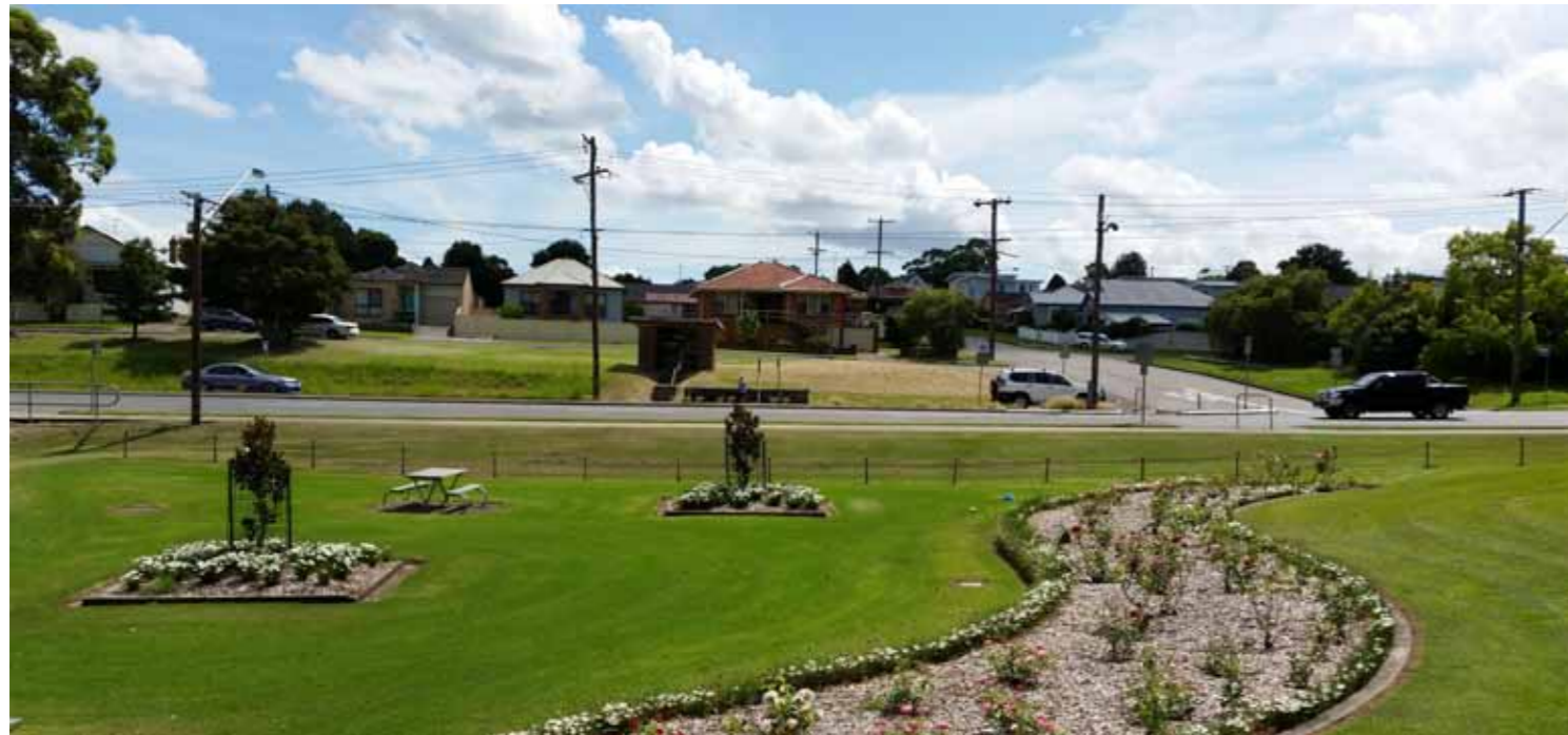
Figure 7.37 View from Jesmond Park looking north towards Newcastle Road and the intersection with Steel Street.
