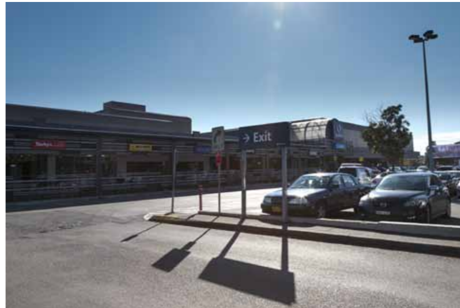
Figure 3.64 Car parks are a dominant feature within this character zone. Lack of greenery and dominant built form elements such as the Stockland Jesmond Shopping Centre define the sense of place.
