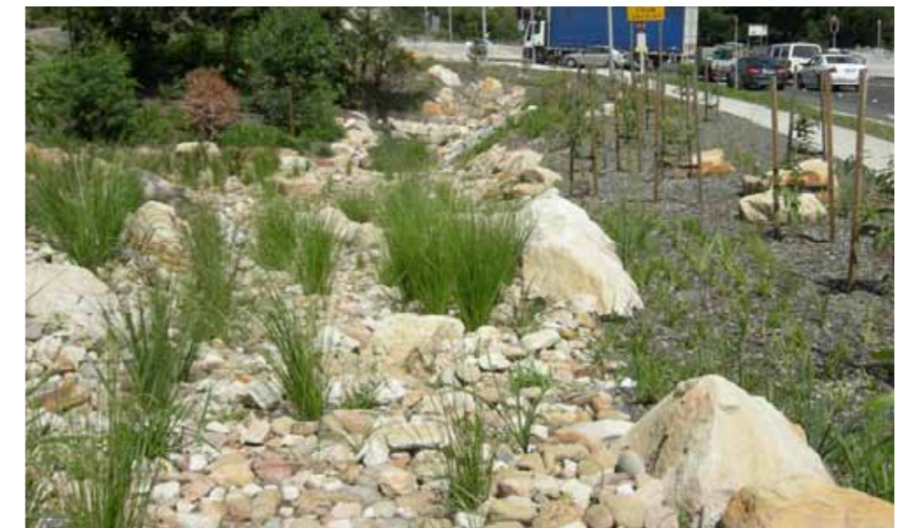
Figure 5.36 Rock mulched swales could be used where velocities are higher, and would be planted with wetland filter plants, similarly to the vegetated swales.
