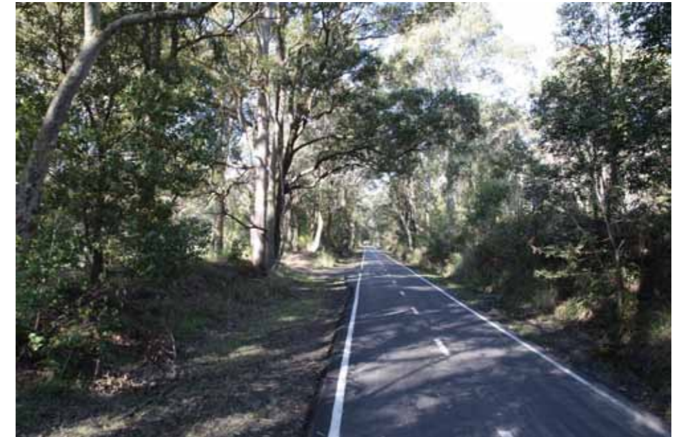
Figure 2.11 Cycle path through woodland area, east of the Northern Interchange.
