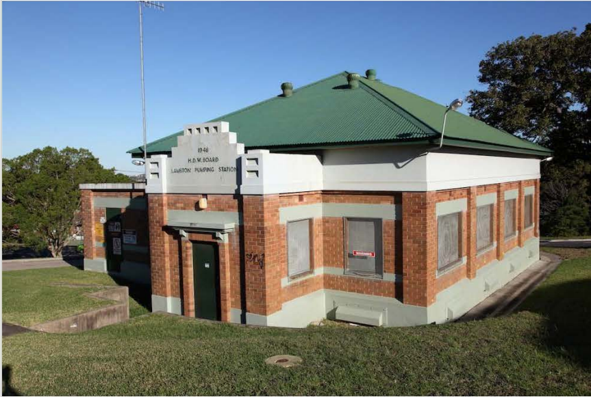
Lambton Water Pump Station
