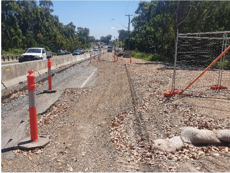
Image 5: Utility relocation works
