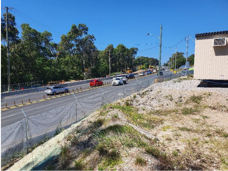
Image 1: Utilities relocation works
