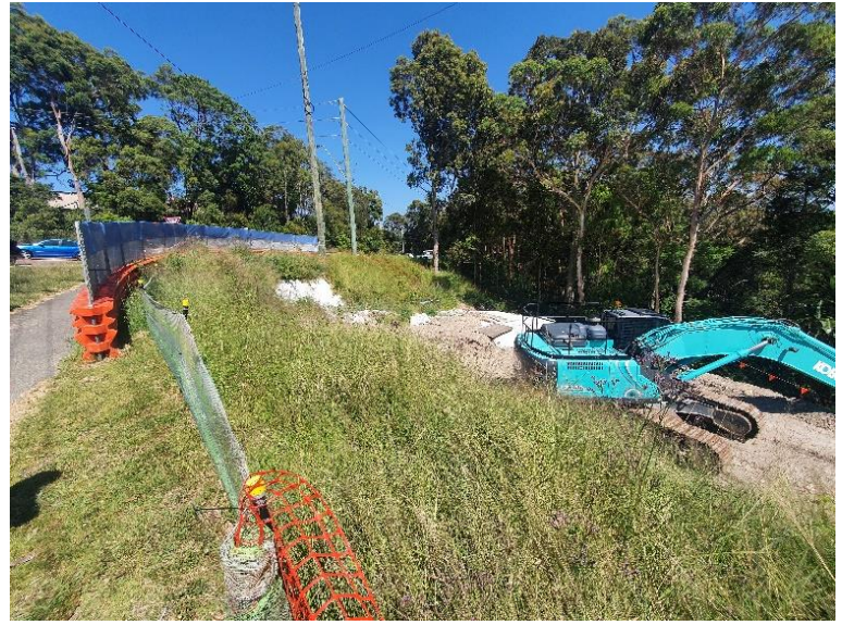
Image 2: Utility relocation works
