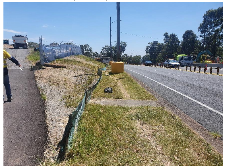
Image 8: Utility relocation works
