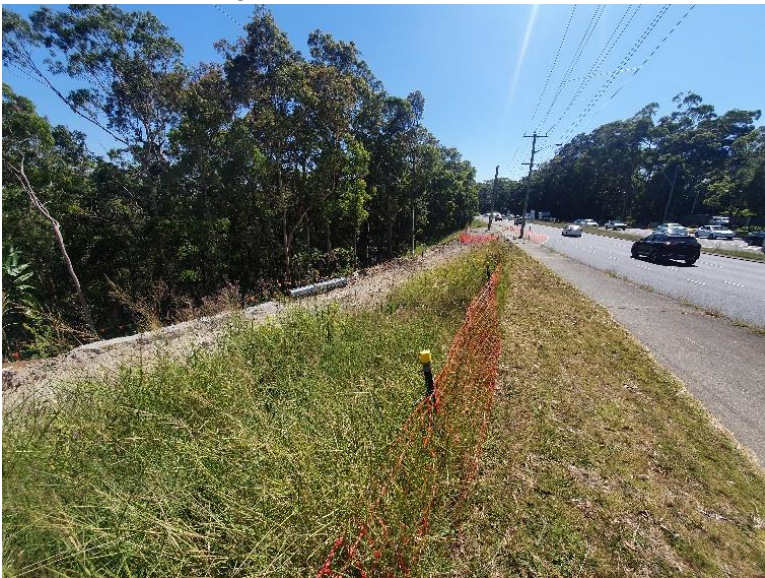
Image 3: Utility relocation works
