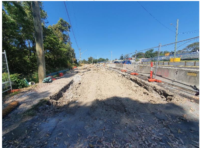
Image 4: Utility relocation works
