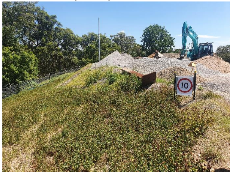
Image 7: Utility relocation works
