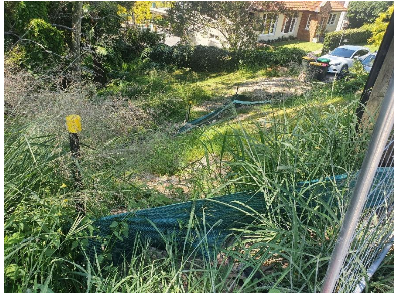
Image 6: Utility relocation works
