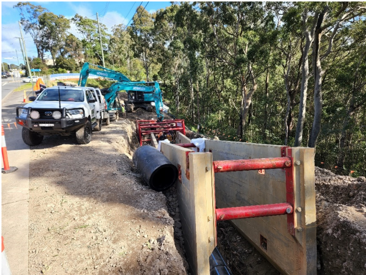
Image 3: Utility relocation works
