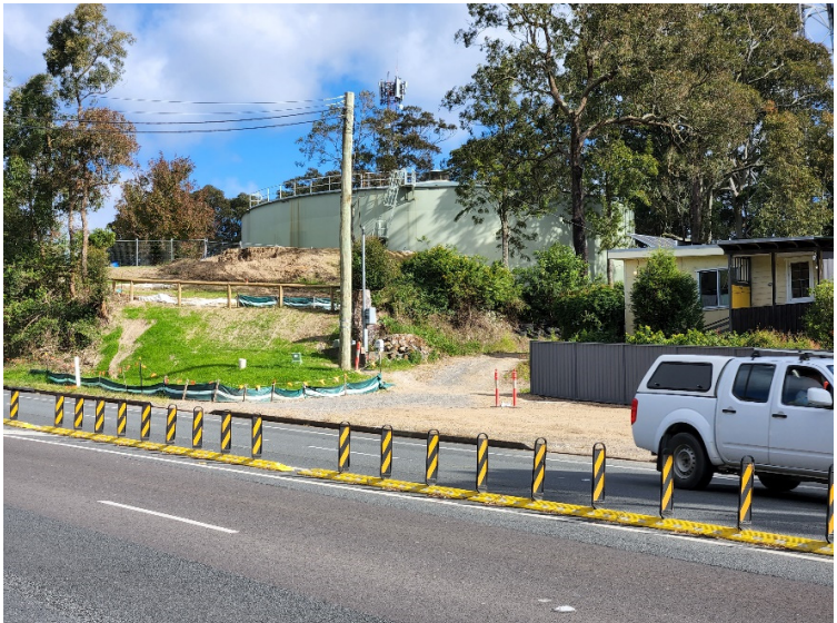
Image 8: Utility relocation works
