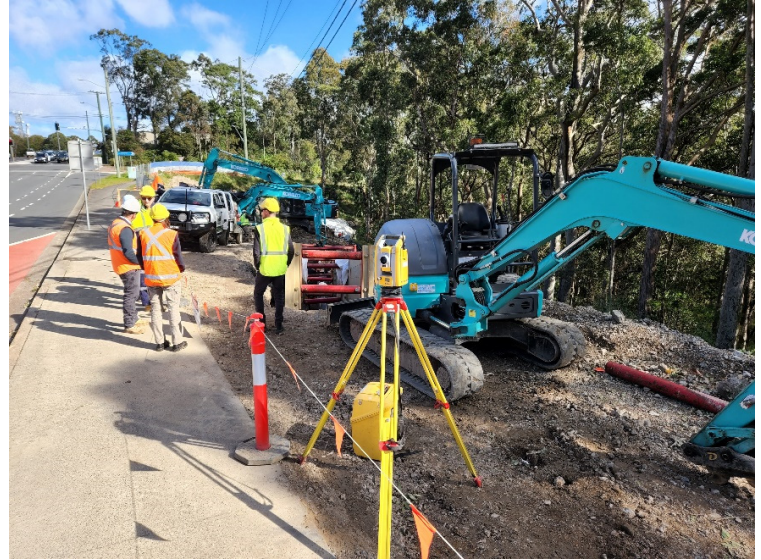
Image 2: Utility relocation works
