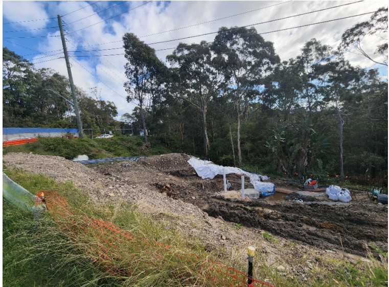
Image 4: Utility relocation works
