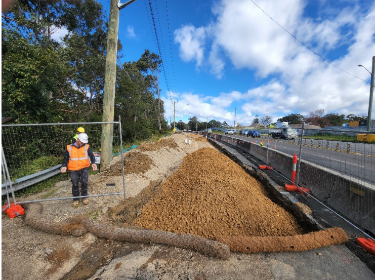
Image 5: Utility relocation works
