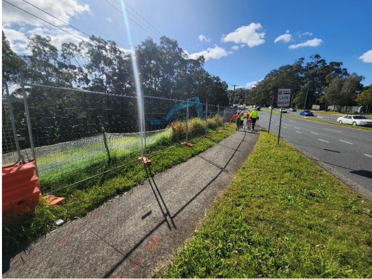
Image 1: Utilities relocation works
