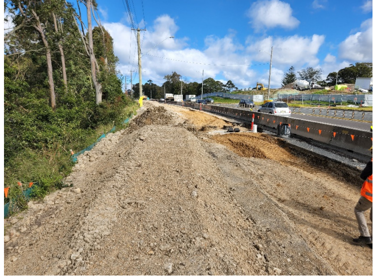
Image 6: Utility relocation works
