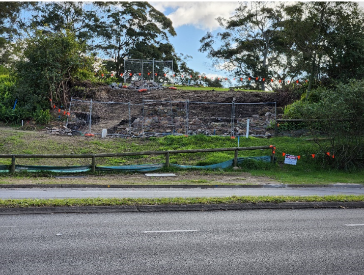
Image 7: Utility relocation works
