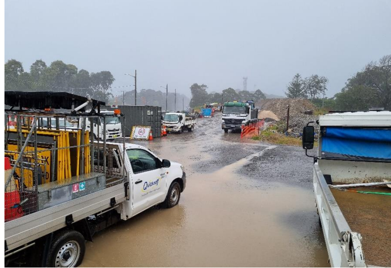
Image 2: Utility relocation works
