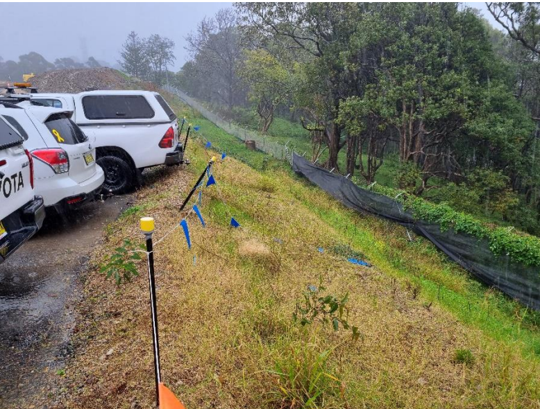
Image 3: Utility relocation works
