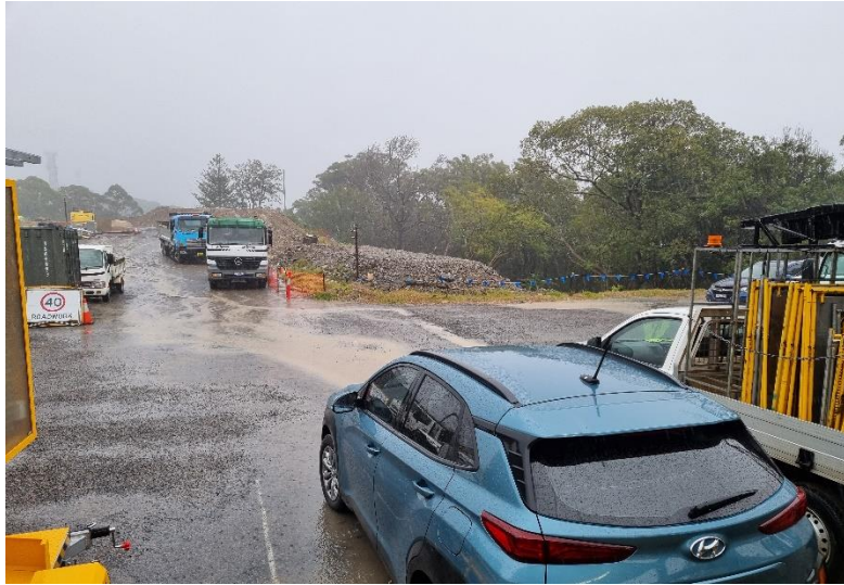
Image 1: Utilities relocation works
