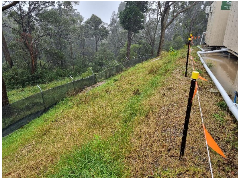
Image 4: Utility relocation works
