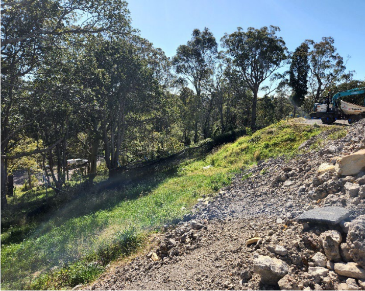
Image 1: Utilities relocation works
