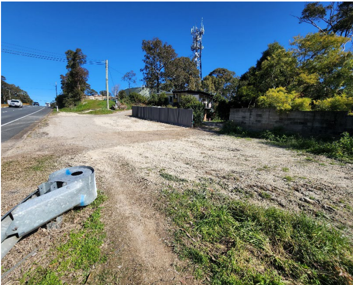
Image 3: Utility relocation works
