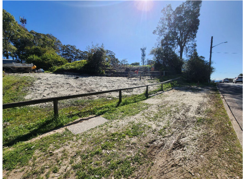
Image 4: Utility relocation works
