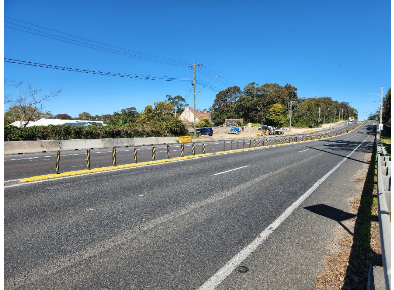
Image 2: Utility relocation works
