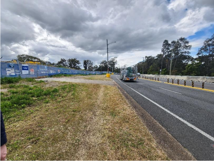
Image 5: Southern utilities relocation works
