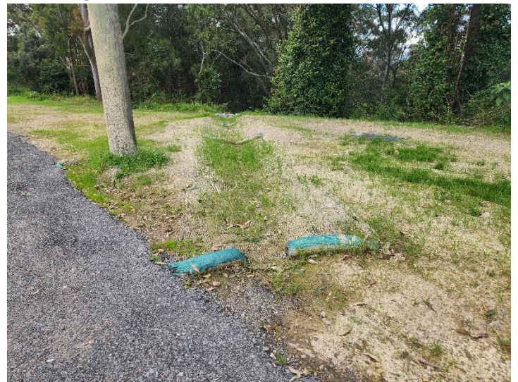
Image 8: Southern utilities relocation works
