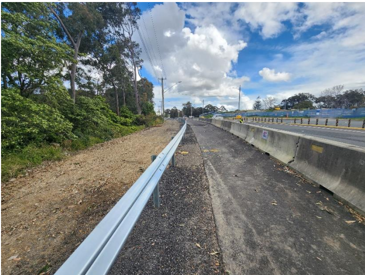
Image 7: Southern utilities relocation works
