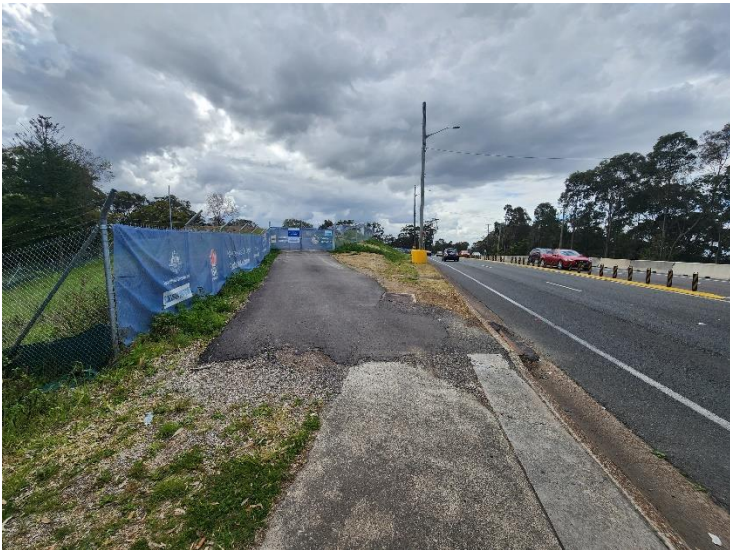
Image 3: Southern utilities relocation works
