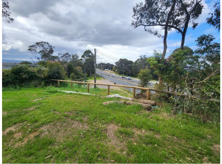
Image 2: Southern utilities relocation works
