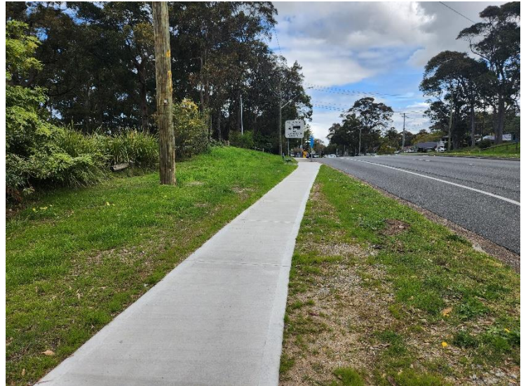
Image 4: Southern utilities relocation works
