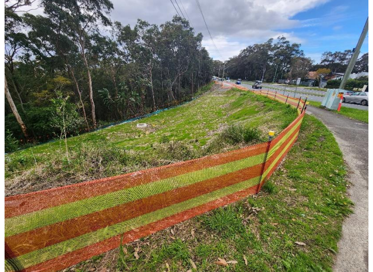
Image 6: Southern utilities relocation works
