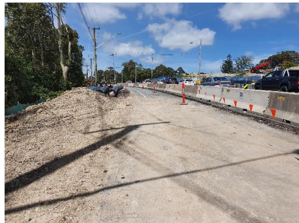
Image 4: Utility relocation works
