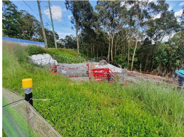
Image 2: Utility relocation works
