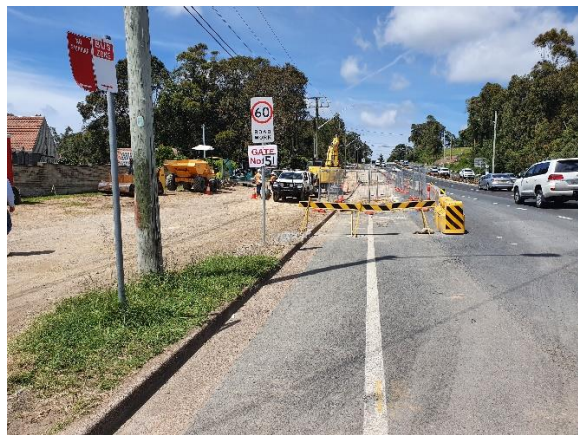
Image 5: Utility relocation works
