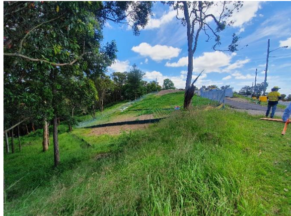
Image 6: Utility relocation works
