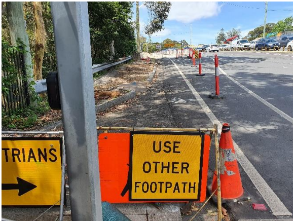
Image 3: Utility relocation works
