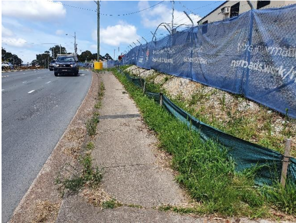
Image 1: Utility relocation works
