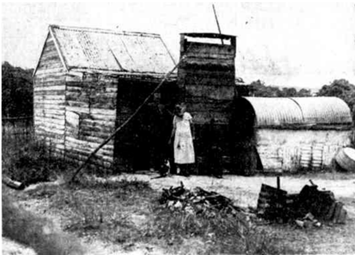
Figure 2.7: An example of a humpy at Hollywood Unemployment Camp in January 1941. This two room iron and timber hut was occupied by a pensioner couple. The curved roof structure on the right, made from halved water tanks, was used as a pantry where they stored vegetables from their garden. Source: Newcastle Sun 24 Jan 1941, p.5.
