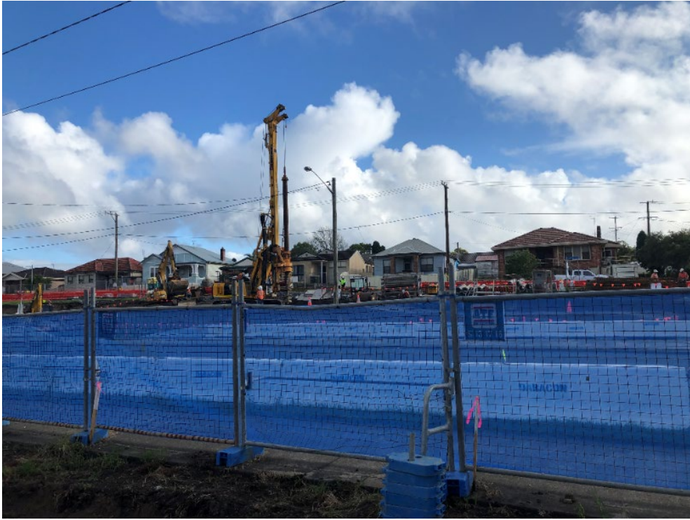
Photograph D.5 Evidence of appropriate fencing surrounding construction works
