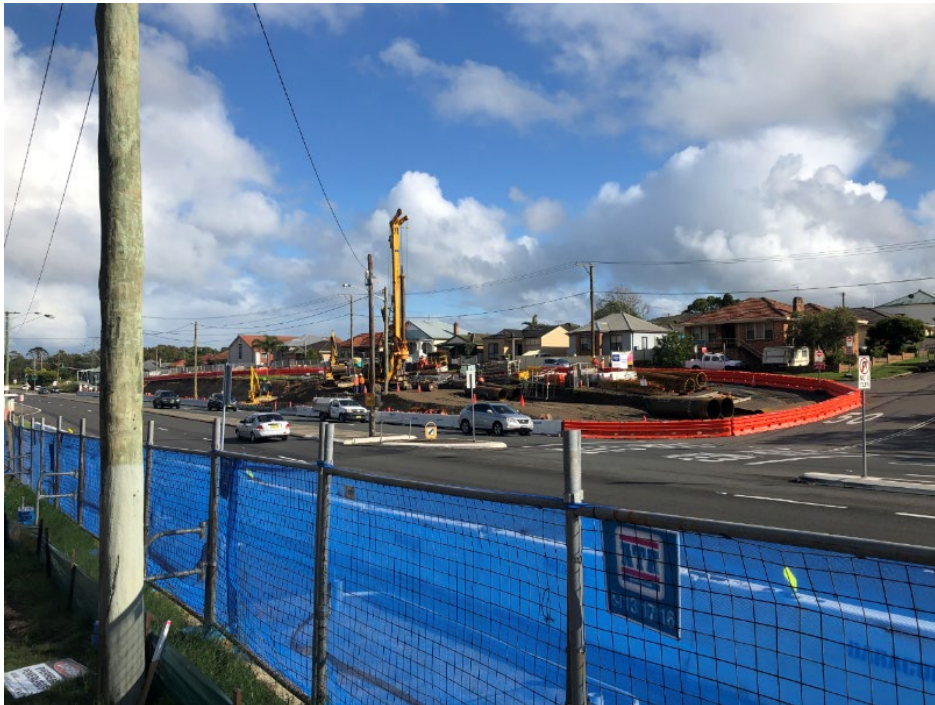
Photograph D.6 View of construction of works along Newcastle Road
