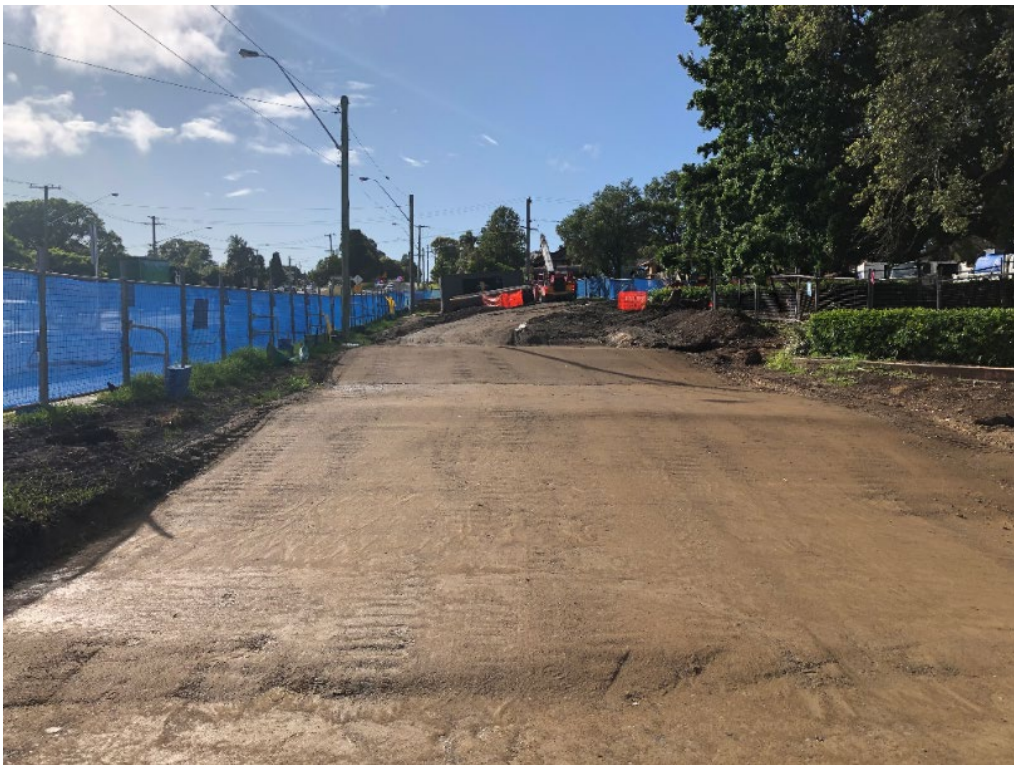
Photograph D.4 View of works associated with road realignment and widening
