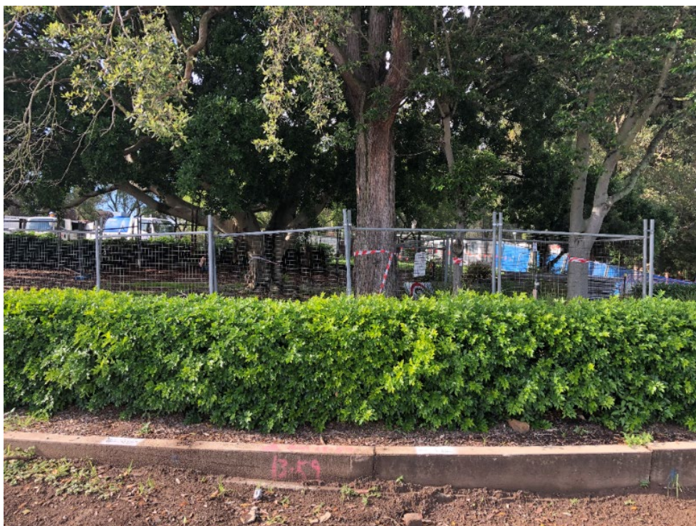
Photograph D.7 Evidence of appropriate fencing around retained trees
