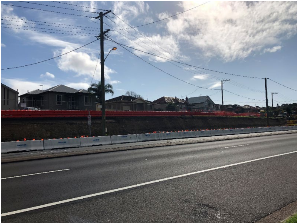
Photograph D.9 View of earthworks along Coles Street and residences
