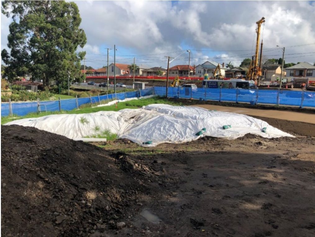
Photograph D.3 Evidence of appropriately covered stockpiling areas
