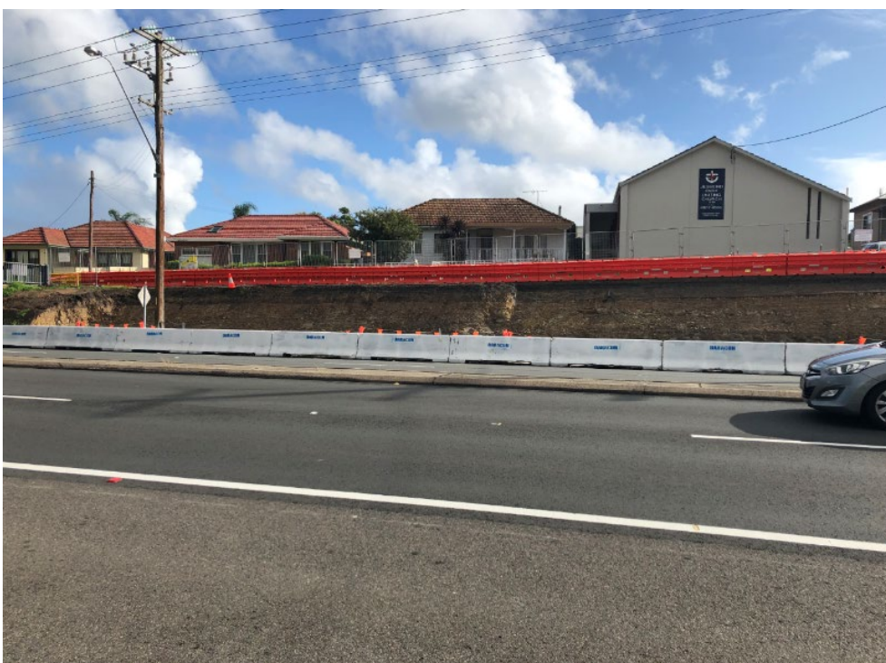
Photograph D.8 Evidence of earthworks and appropriate signage and access controls for pedestrian, cyclists and vehicle access
