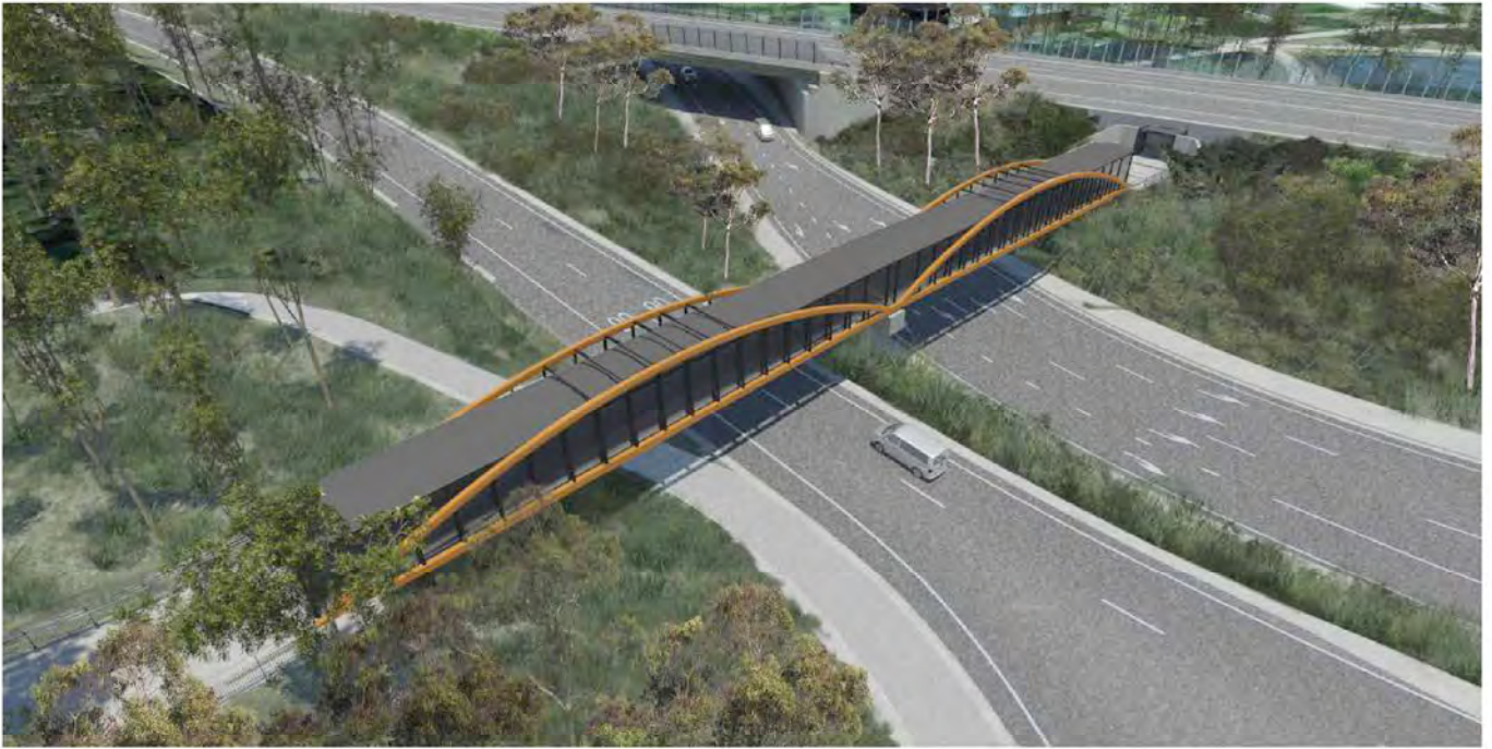
Indicative 3D image of Bridge 8 - shared path bridge at northern interchange, looking south
