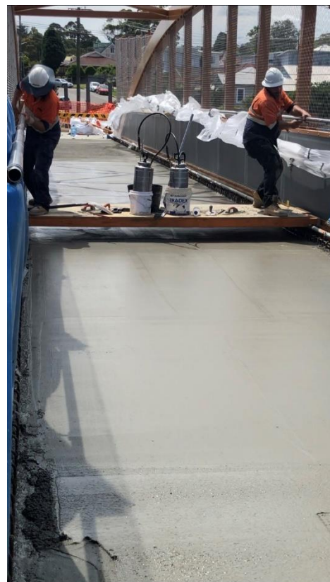
Image 7: Railed timber deck in operation
