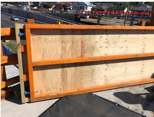
Image 6: Railed timber deck for concreting bridge deck
