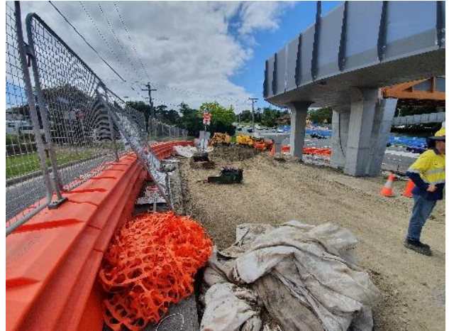
Image 5: Northern works, Newcastle Road
