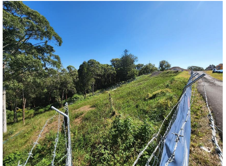
Image 4: Utility relocation works
