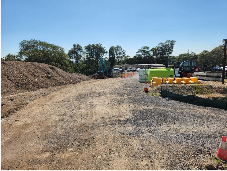
Image 1: Utilities relocation works
