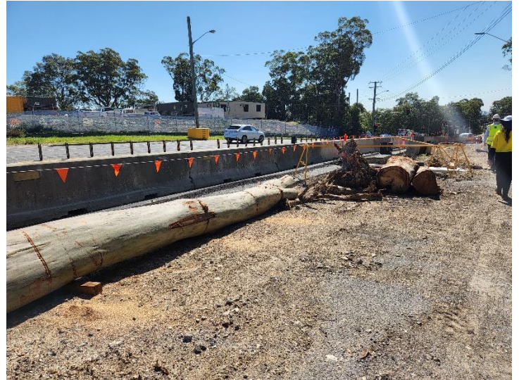
Image 8: Utility relocation works
