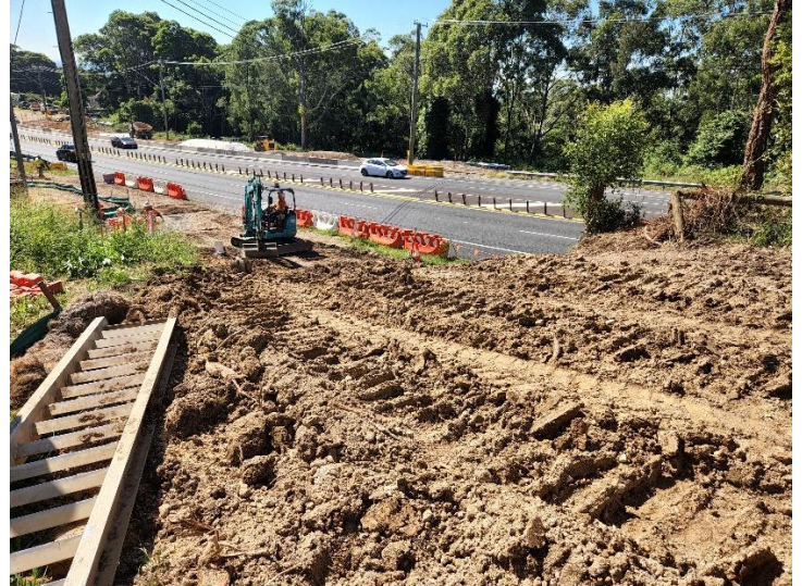
Image 6: Utility relocation works
