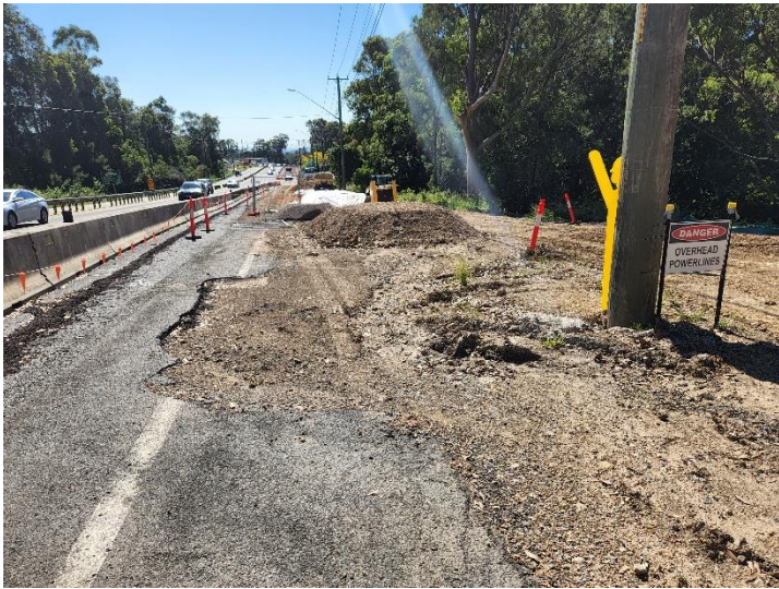
Image 7: Utility relocation works
