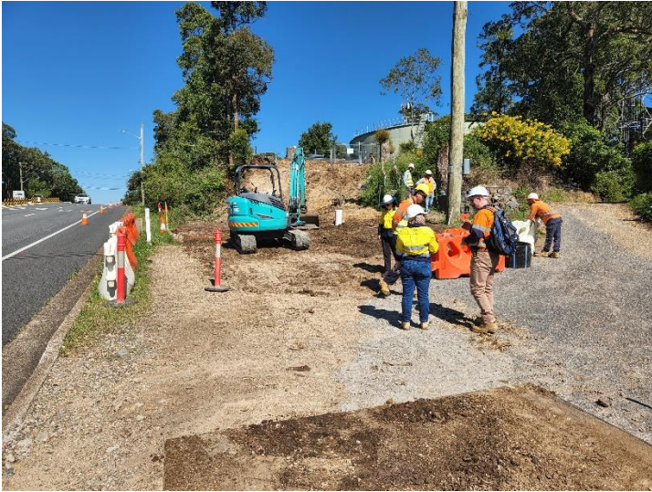
Image 5: Utility relocation works
