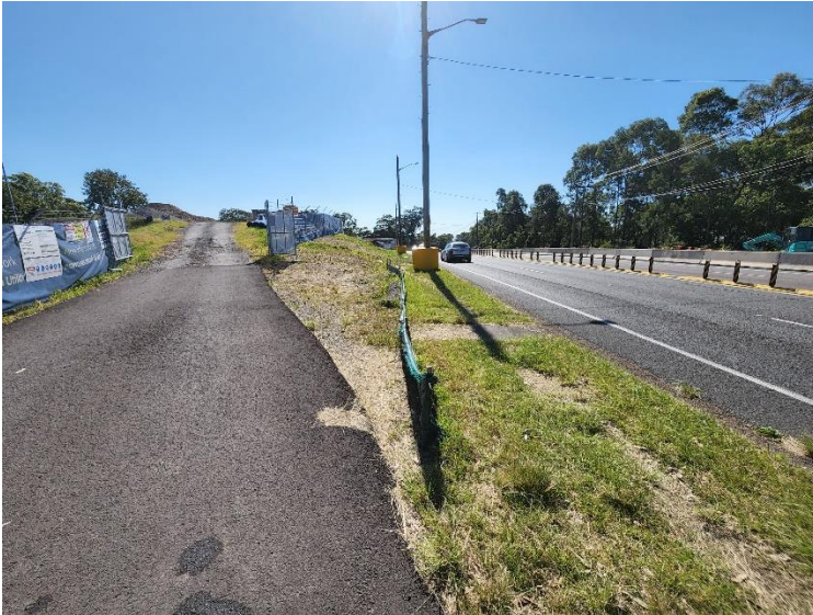
Image 3: Utility relocation works
