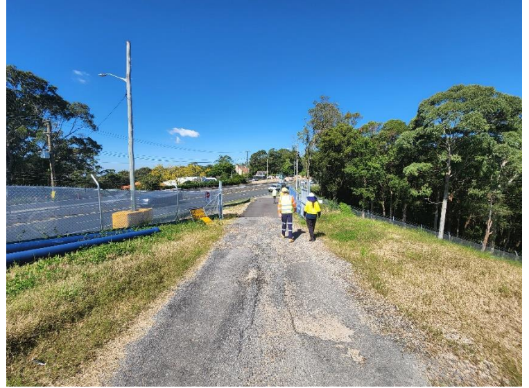
Image 2: Utility relocation works
