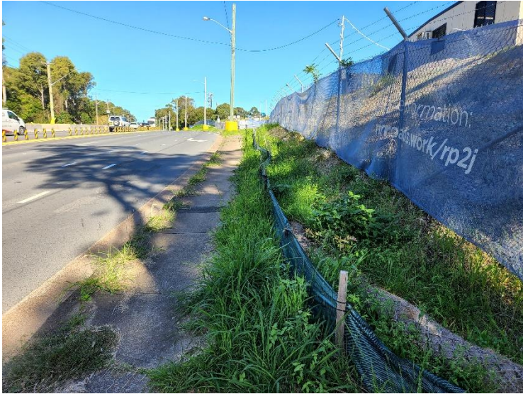
Image 1: Utilities relocation works
