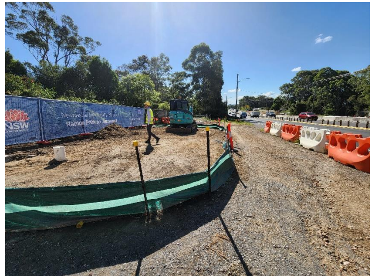
Image 8: Utility relocation works
