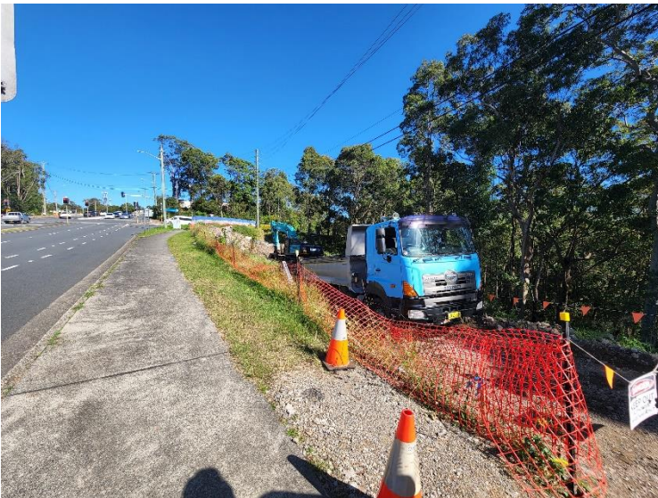
Image 3: Utility relocation works
