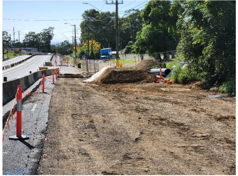
Image 6: Utility relocation works
