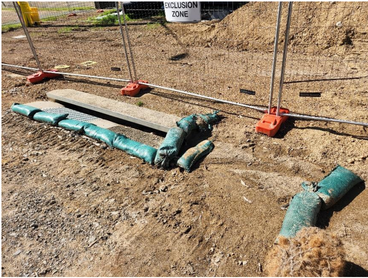
Image 5: Utility relocation works
