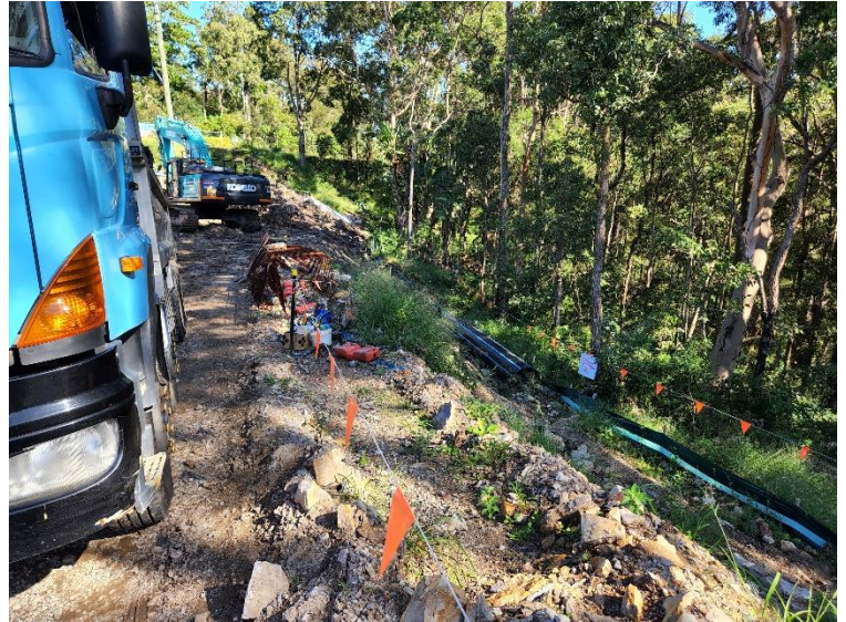
Image 2: Utility relocation works
