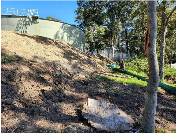
Image 7: Utility relocation works
