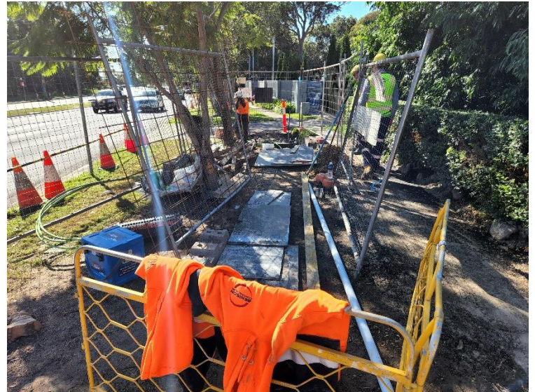
Image 4: Utility relocation works
