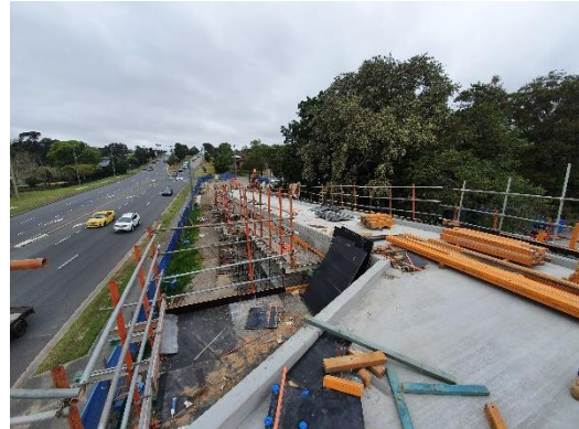
Image 2: Southern Bridge Access Ramp
