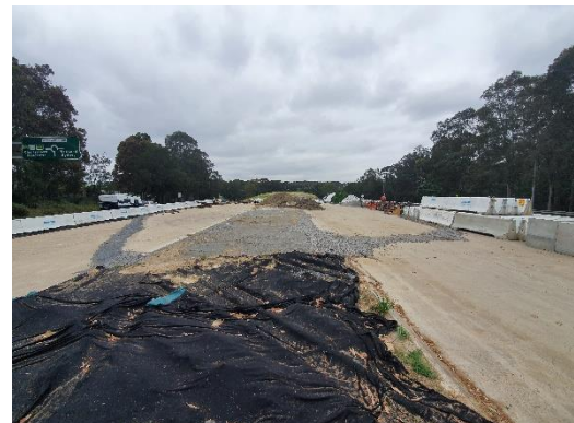
Image 6: Storage Area, Main Road
