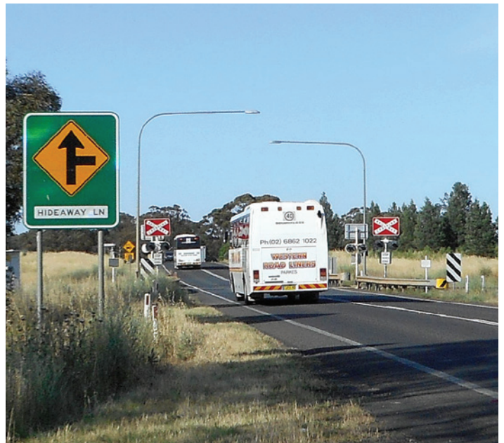
Newell Highway at the Welcome railway crossing
