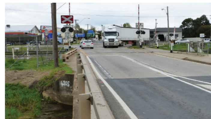
Truck turning over the level crossing from Hartigan Avenue
