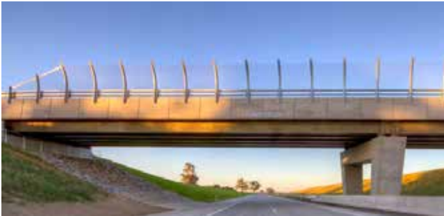
Figure 78 Throw screens matched to the spacing of the parapet panels.
