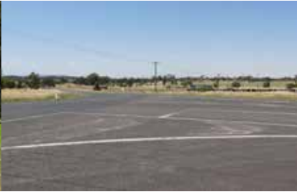
Figure 7 - Location of bridge crossing (Hartigan Avenue)
