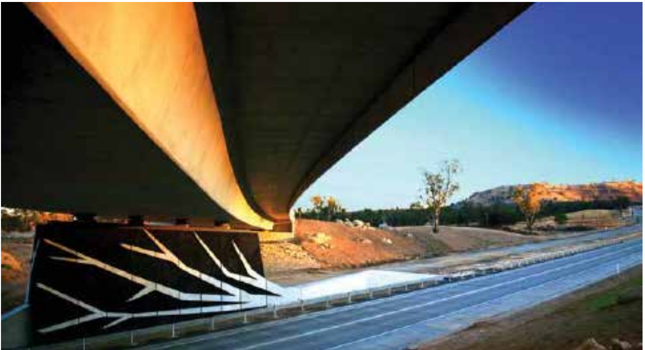
Figure 75 - Lizard Tree - Tumbarumba Bridge Pier, Hume Highway - Jackson Teece
