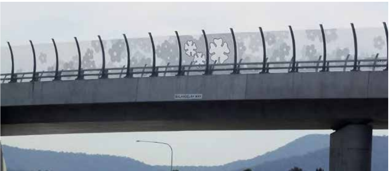
Figure 79 Artwork integrated into the mesh panels on the Bulahdelah access bridge fence design. Source: Achievements in Roads and Maritime Services Infrastructure Projects. (Roads Services)
