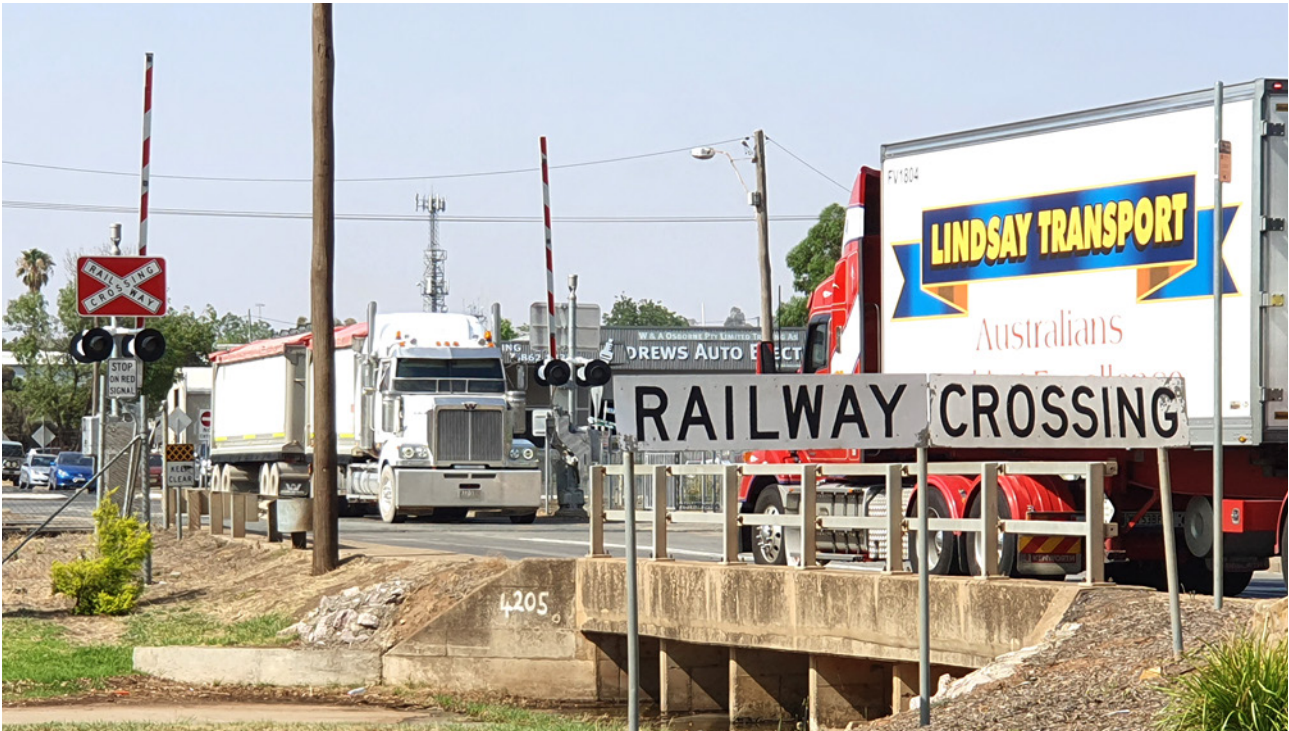
Heavy traffic on the Newell Highway railway crossing in Parkes
