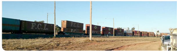
The bridge over the Broken Hill and Parkes to Narromine rail lines at Hartigan Avenue will accommodate double stacked container trains
