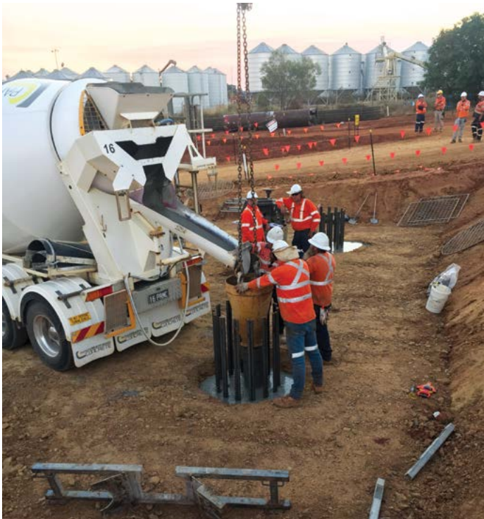
Piling for the Bridge over Rail and Hartigan Avenue
