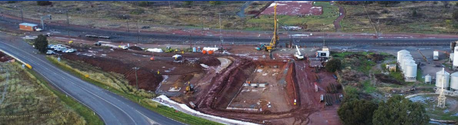
Hartigan Avenue and Billy Mac Place intersection
