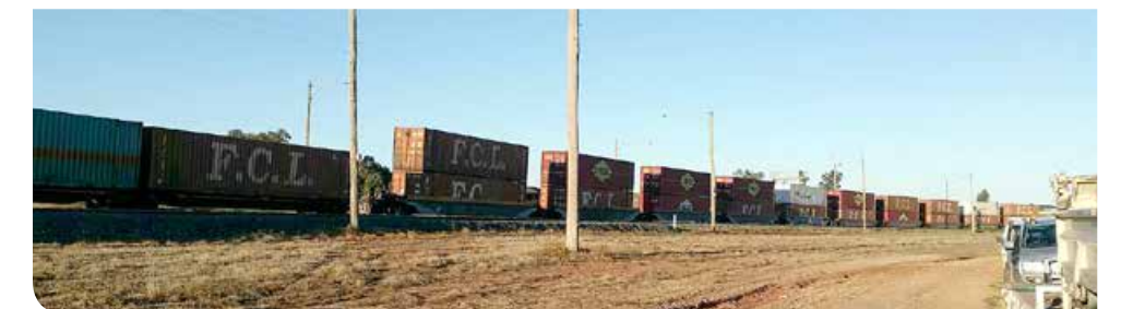
The bridge over the Broken Hill and Parkes to Narromine rail lines at Hartigan Avenue will accommodate double stacked container trains
