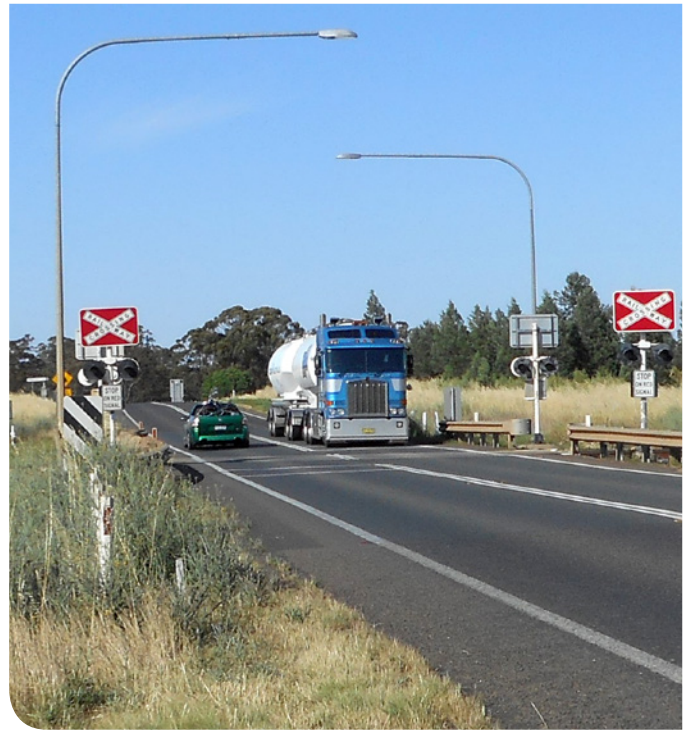
Newell Highway at the Welcome railway crossing south of Parkes
