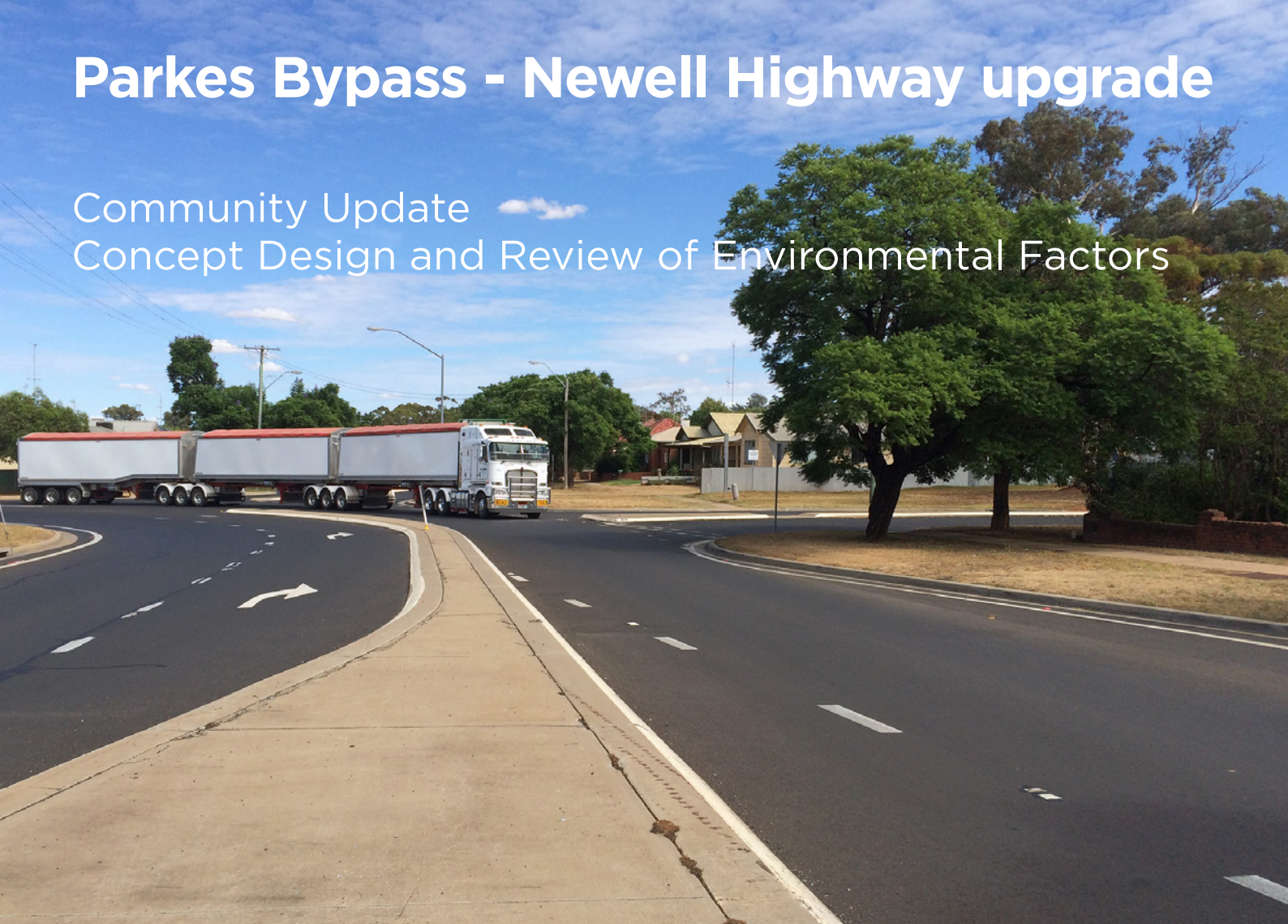
A PBS3a vehicle struggling to negotiate the existing Newell Highway through Parkes
