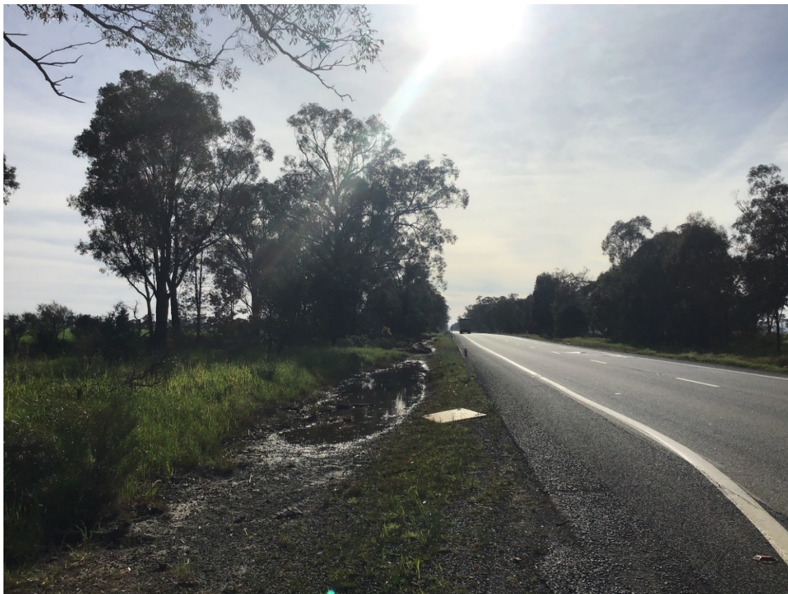
Photo 5-1 Existing highway showing narrow road shoulders, broken white dividing line and no drainage infrastructure
