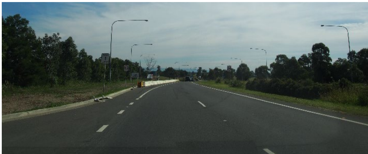
Figure 40 – Views from Richmond Road looking west from Elara Boulevard
