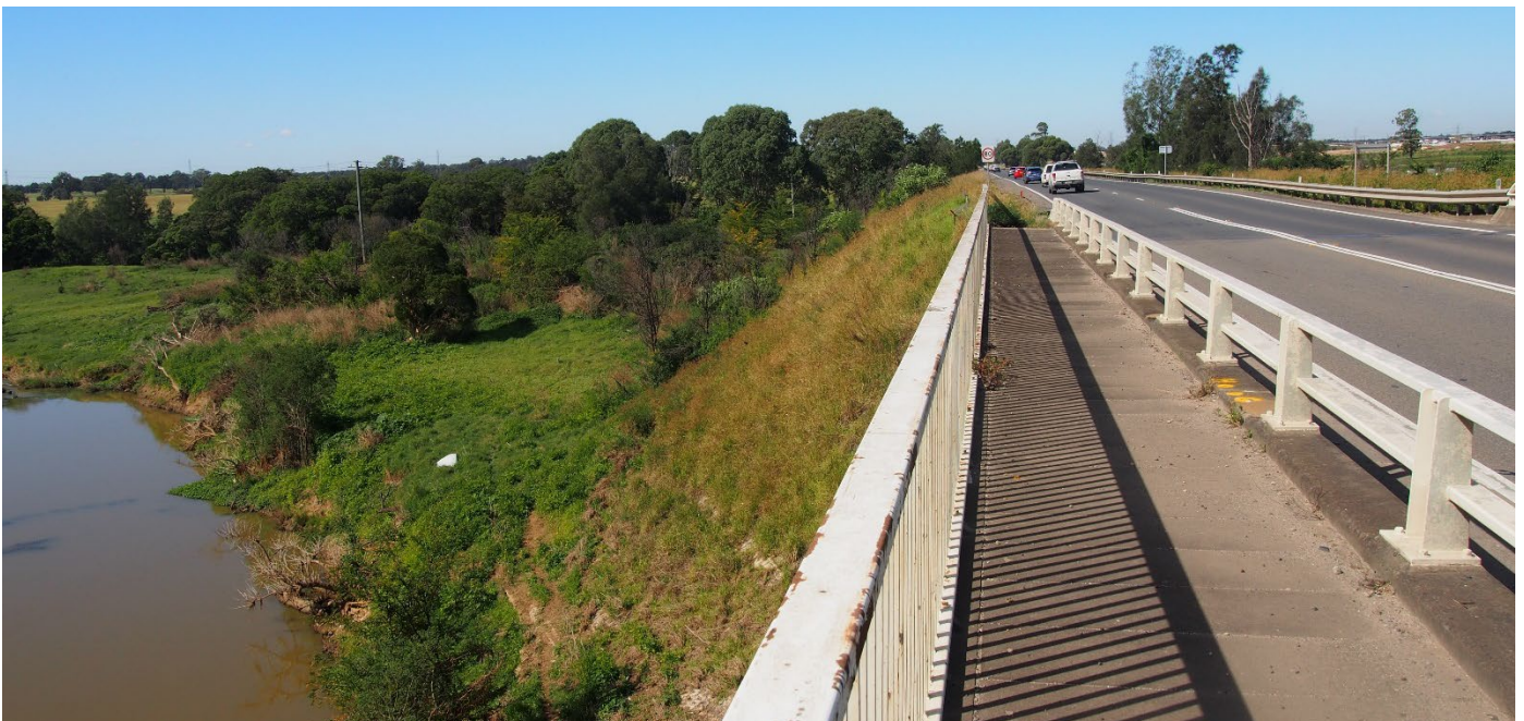
Figure 14 – View from South Creek Bridge looking east
