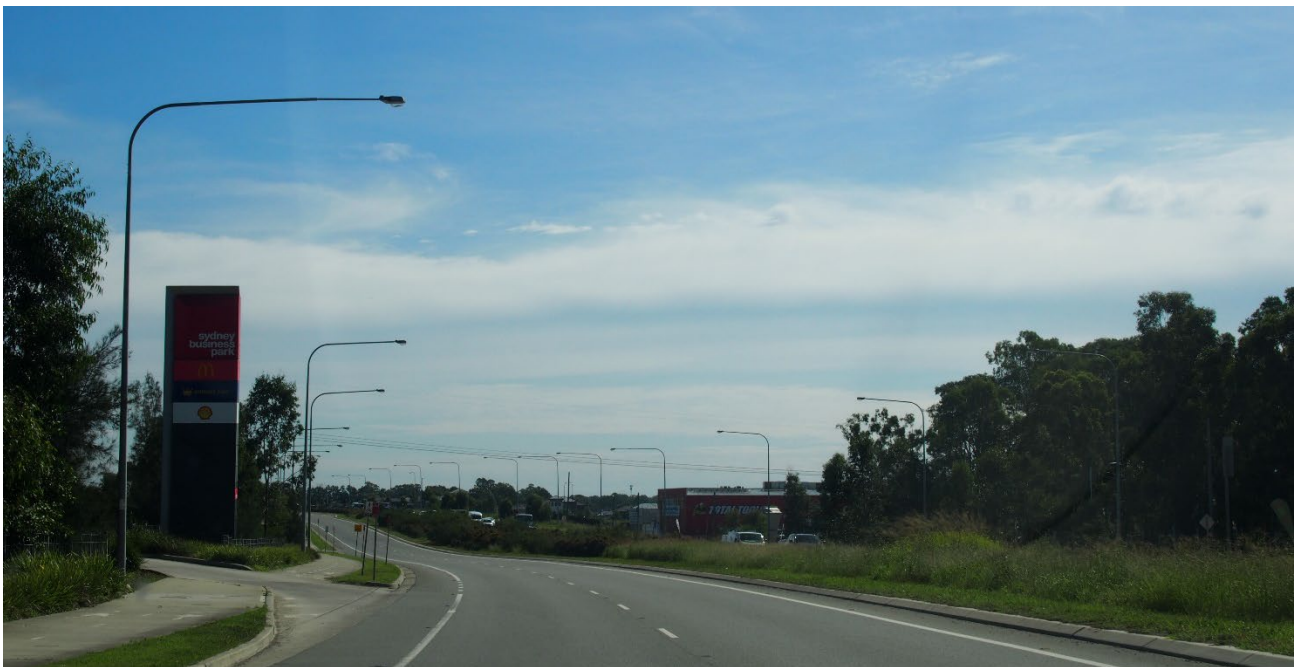
Figure 24 – View of Richmond Road showing typical lighting layout after previous upgrades
