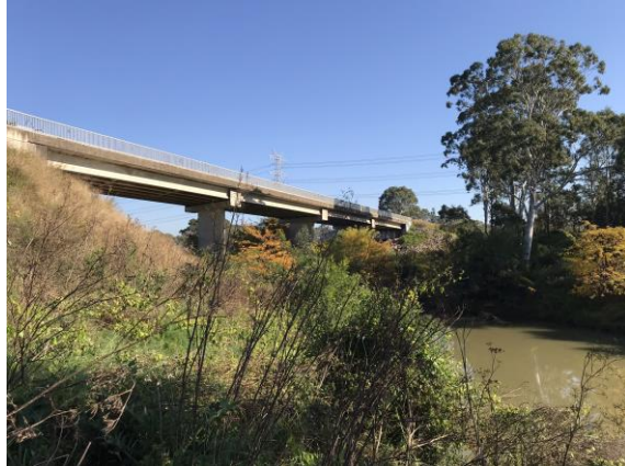
Figure 34. South Creek Bridge from eastern side of Richmond Road, northern aspect
