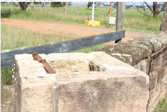
Figure 22. Sandstone wall with coping removed, detail
