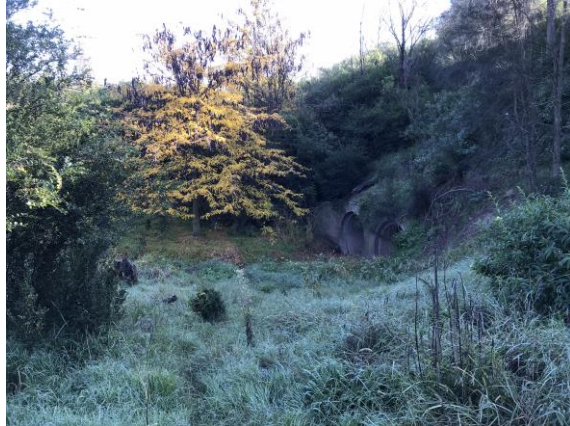
Figure 32. Embankment and culverts under South Creek Bridge, northern aspect
