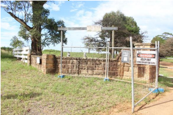
Figure 22. Sandstone wall with coping removed, detail
