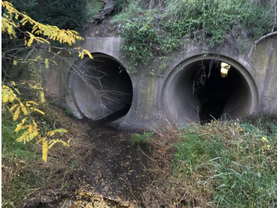
Figure 33. C.1980s culverts beneath Richmond Road, north-eastern aspect
