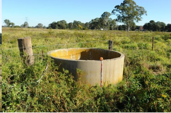
Figure 7. 20th century fence line and aggregate concrete water tank
