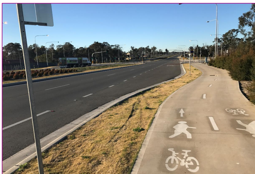
Figure 6: Shared footpath along Richmond Road western carriageway, August 2017
