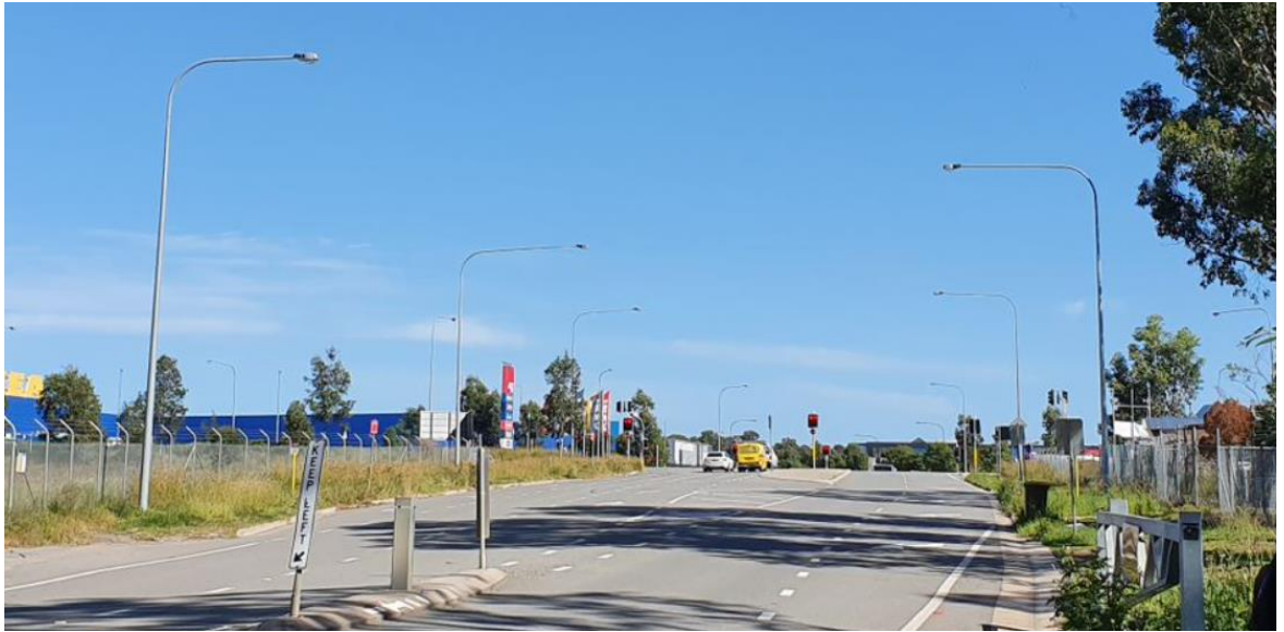
Figure 5.18 Existing LED lighting
