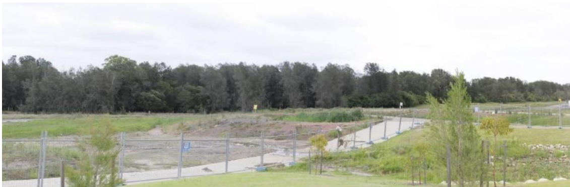
Photo 6 View from Aerodrome Drive (Veron Road) looking north-west
