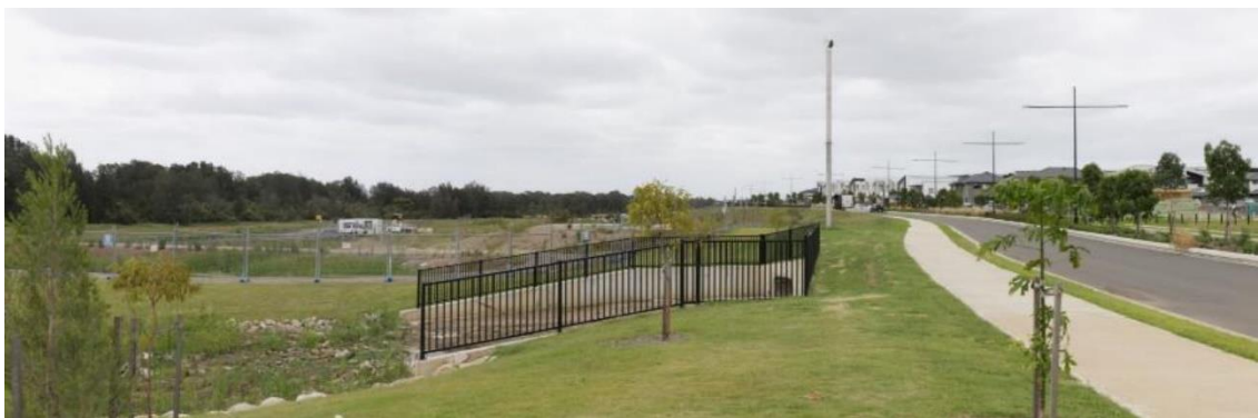
Photo 7 View from Aerodrome Drive (Veron Road) looking north
