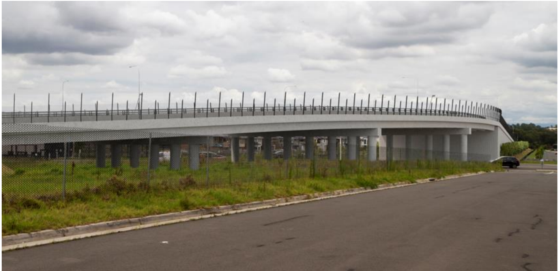
Figure 5.13 Artistic impression showing the rail overbridge from Stoke Street, looking south-west (NTS)
