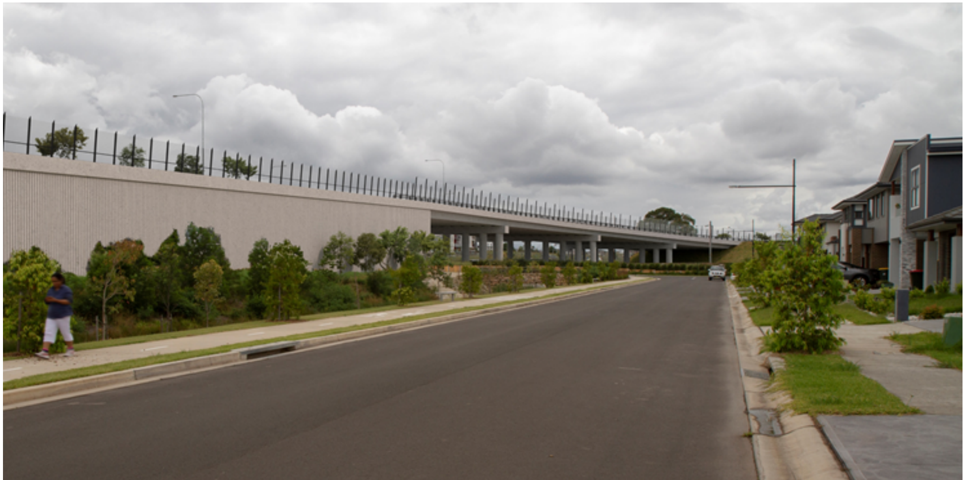
Figure 5.14 Artistic impression showing the rail overbridge from Anson Street, looking north-east (NTS)
