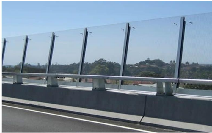
Figure 5.4 Image of vertical safety screen with highly visual permeability and indicative cross section
